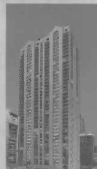
Towering opportunity: 200 North Dearborn Private Residences, a 47-story luxury high-rise, offers a prime location in Chicago's Loop. ↑ SUPPLIED PHOTO
