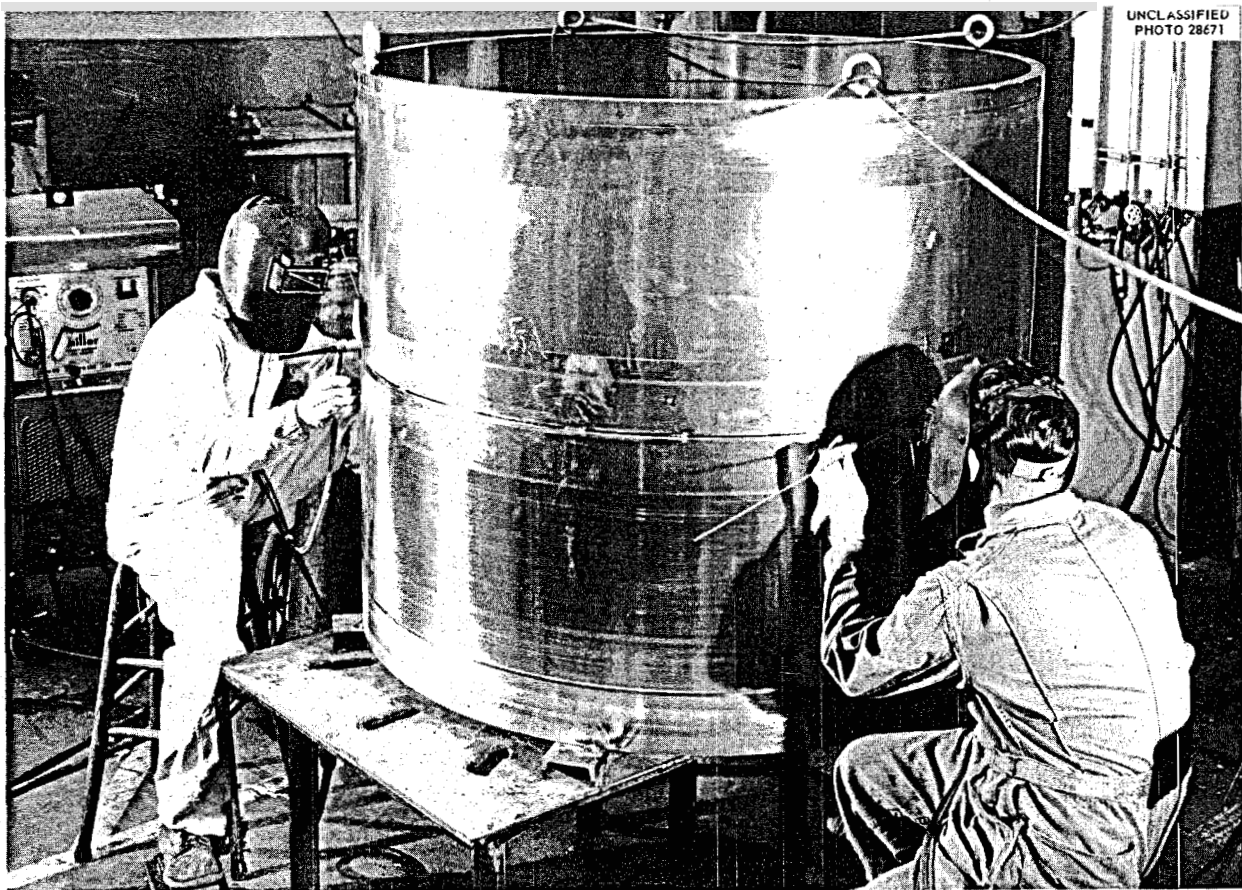
Fig. 1.1.1. Pressure Shell Weld Test.
