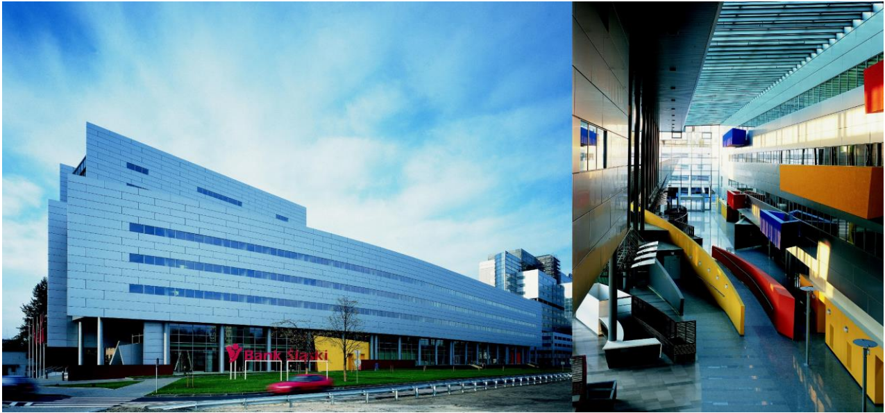
Fig. 2. 'Hull' facade and 'lifeboat' balconies in the Bank Śląski building in Katowice; source: author's archives
