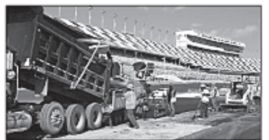
Daytona Superspeedway being repaved to repair potholes that delayed last year's Daytona 500. Michigan International Speedway has announced a preemptive repaving plan to avoid a similar situation. (NASCAR photo)
