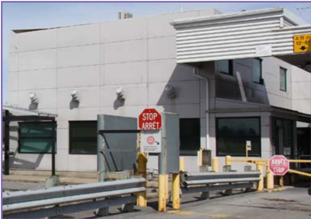
A community plebiscite will be held on April 26, 2014 to gather the community's opinion on the future of several buildings located within the Kawehno:ke corridor that once served as the former-Canada Customs and the Akwesasne Peoples Fire.
