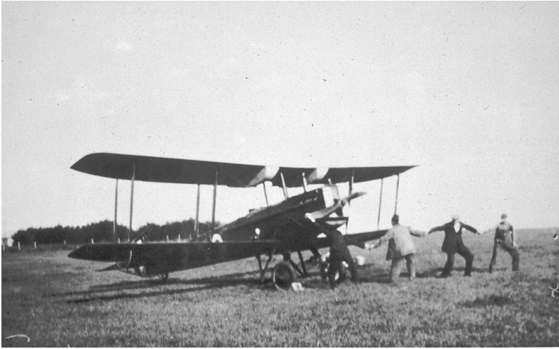
Figure 9 Avro Viper 552A at High River in ca. 1926. Station personnel are hand chain starting the Viper (source: Glenbow Museum NA-2097-17).
