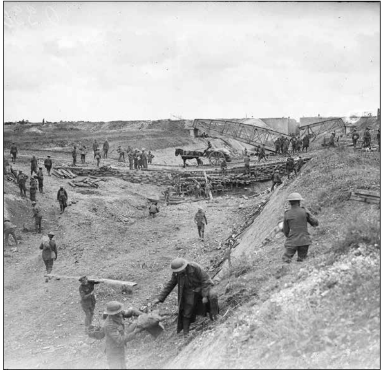
Canadian transport moves across makeshift bridges constructed in the dry bed of the Canal du Nord.
