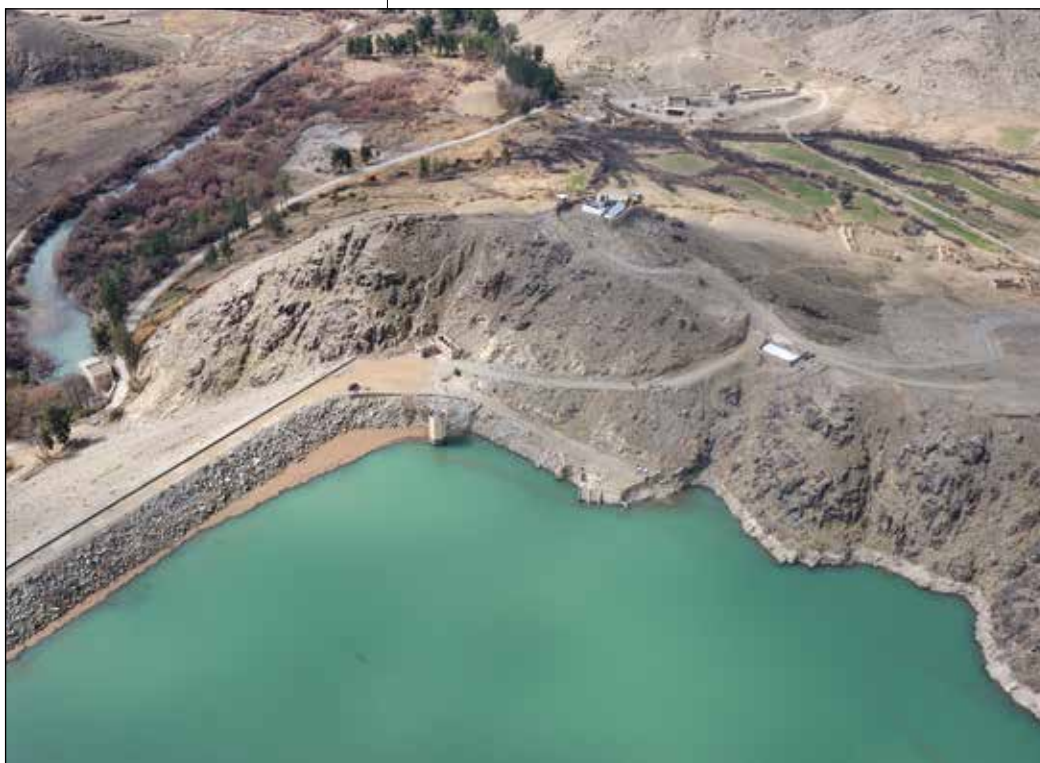
The Dahla Dam and irrigation system, one of three Canadian signature projects in Afghanistan.
