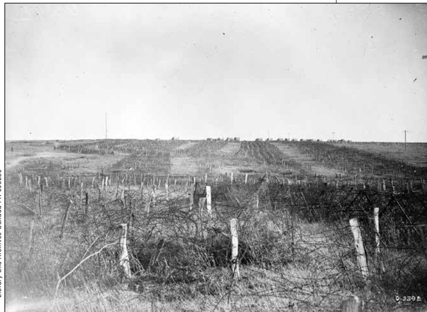
Belts of barbed wire protecting the Hindenburg Line.
