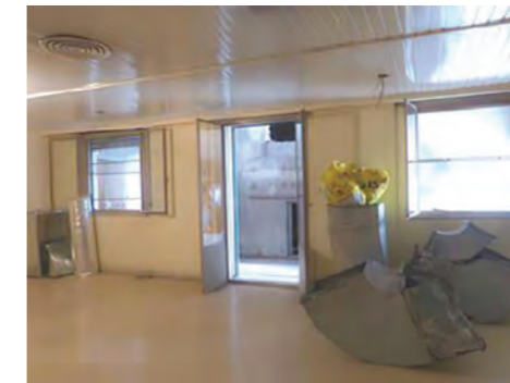
Heating and air conditioning installation: cleaning and partial renovation of the air ducts for its reuse, and placement of new devices. (Source: Martín Capeluto / MSME)
