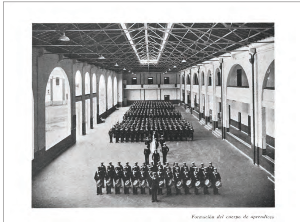
Cadets in formation in the Central Pavilion of the Navy School of Mechanics. (Source: Revista de Arquitectura , SCA, N.º 98, 1928)
