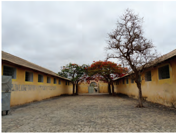
Internal yard in the Tarrafal Concentration Camp, in 2009. (Source: F. Mira)
