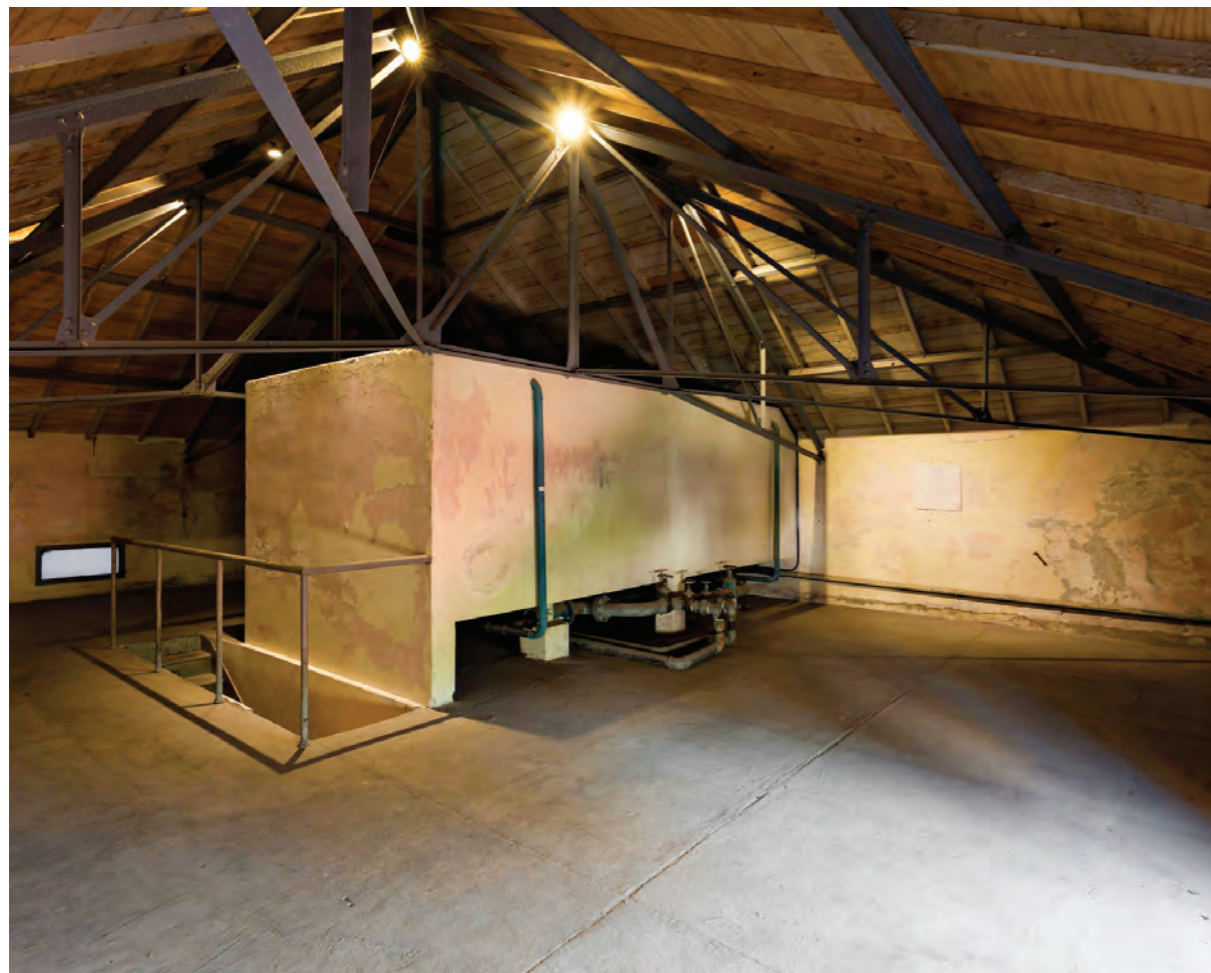
Cement water tank located in Capuchita (Little Hood). (Photo 47: Camilo del Cerro / MSME)
