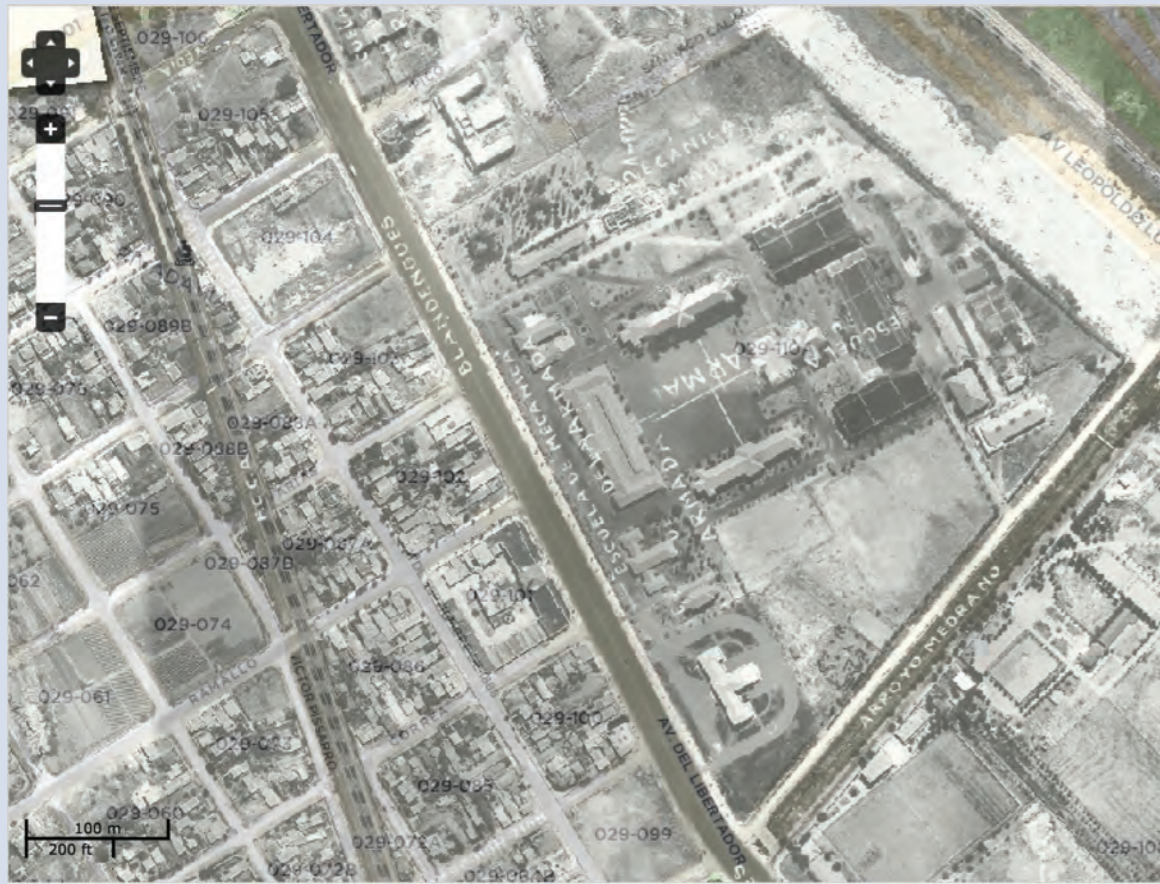
Aerial photo of the property of Navy School of Mechanics (1940). Located on the bordering lot to the NW, one can see the Teachers' Residence. (Source: Undersecretariat for Records, Interpretation and Cadastre, Ministry of Urban Development and Transport, Government of the Autonomous City of Buenos Aires)
