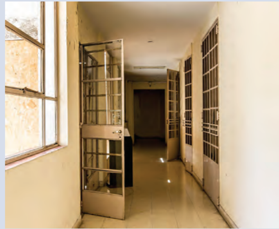
Enclosure of the North and South galleries carried out before IACHR's visit in 1979. (Photo 48: Camilo del Cerro / MSME)
