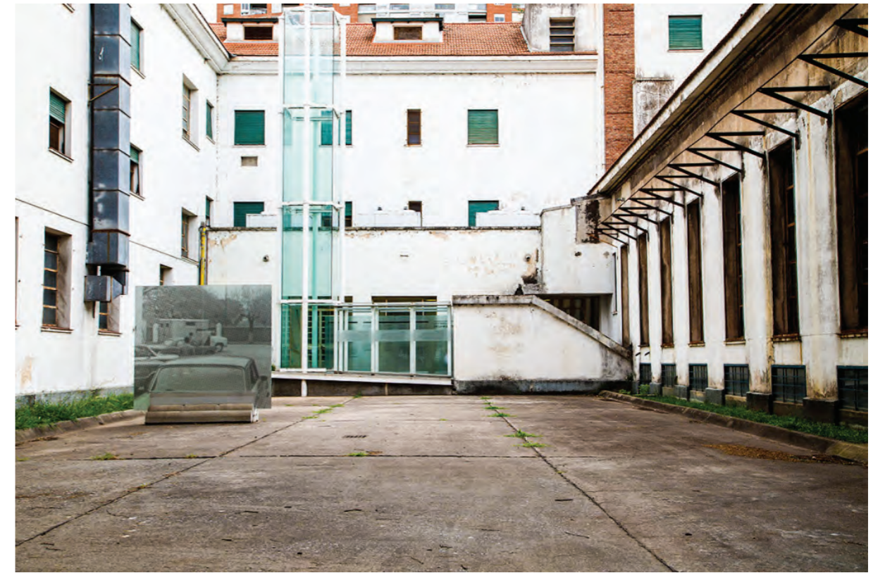
Rear view of Transfers Room . (Photo 33: Camilo del Cerro / MSME)
