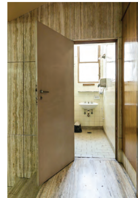
Shaft corresponding to the removed elevator. (Photo 11: Camilo del Cerro / MSME)
