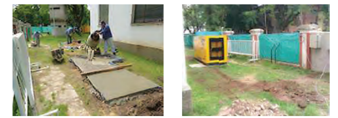
Concrete slab for the placement of the emergency power electric generator. (Source: Martín Capeluto / MSME)
