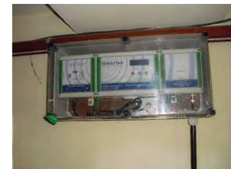
Electro osmotic system for rising damp control, installed in the Basement Level. (Source: Martín Capeluto / MSME)
