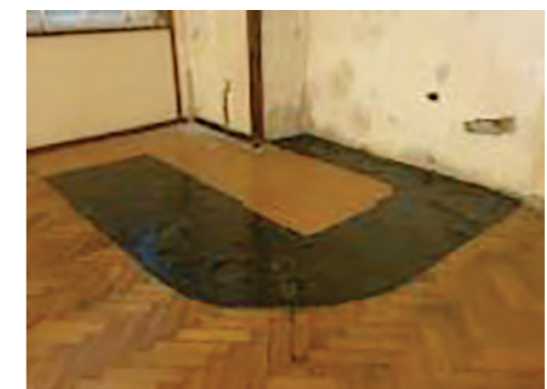
Flooring: before and after cleaning and repair of missing parts procedures on the parquet flooring. (Source: Martín Capeluto / MSME)
