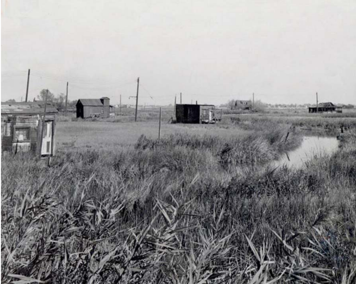
Figure 7. Typical Surface Conditions Within Marine-Tidal-Marsh Areas Prior to Construction of JFKIA [photo credit: Downer, Green and Carrillo].
