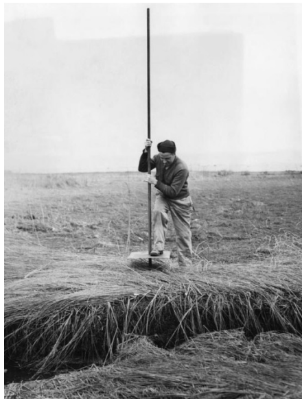
Figure 9. Settlement Plate Placement Prior to Hydraulic Filling.
