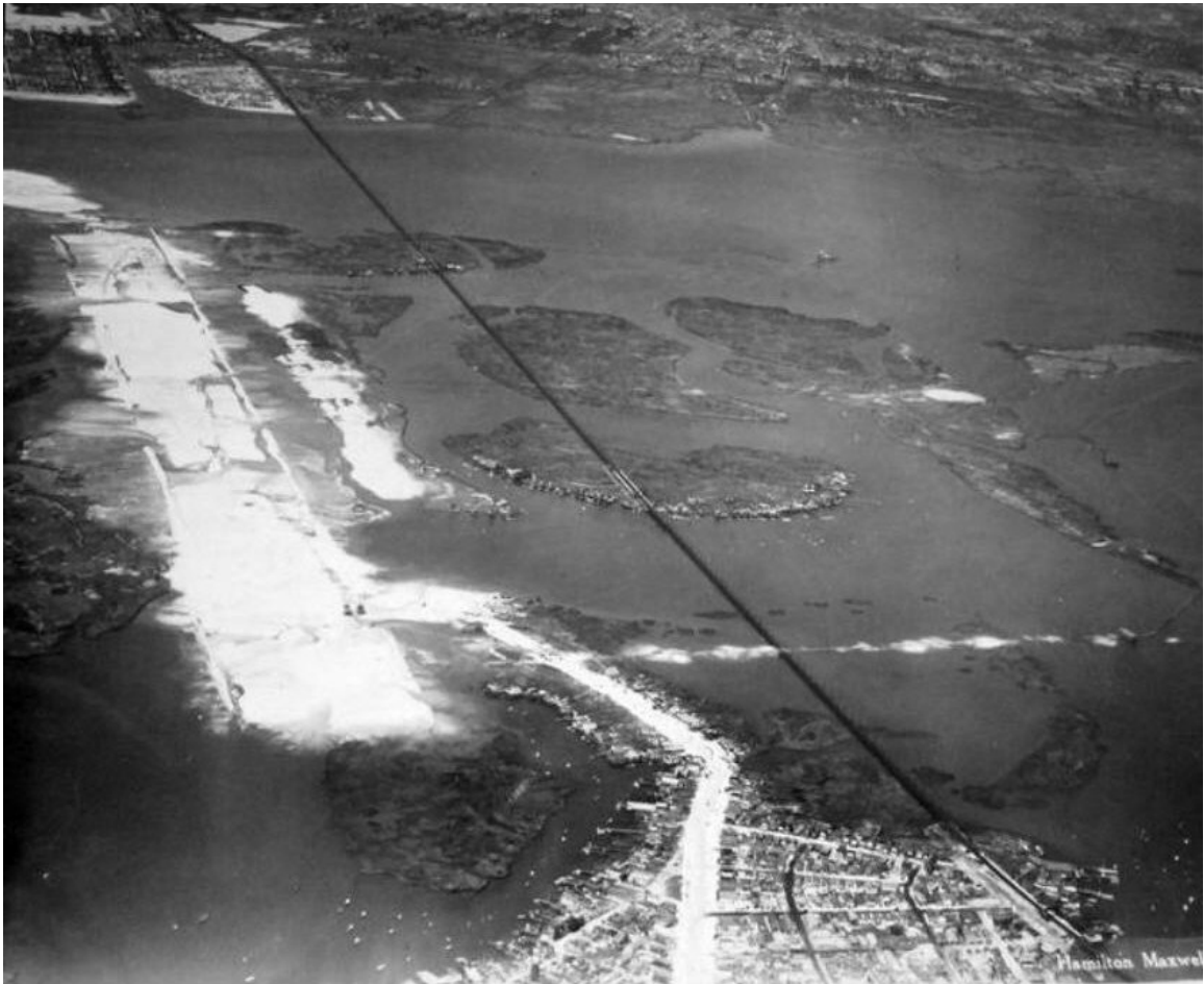
Figure 8. Circa Early-1920s Aerial Photograph Showing Hydraulic Filling for Embankment Portions of Cross Bay Boulevard Under Construction.
