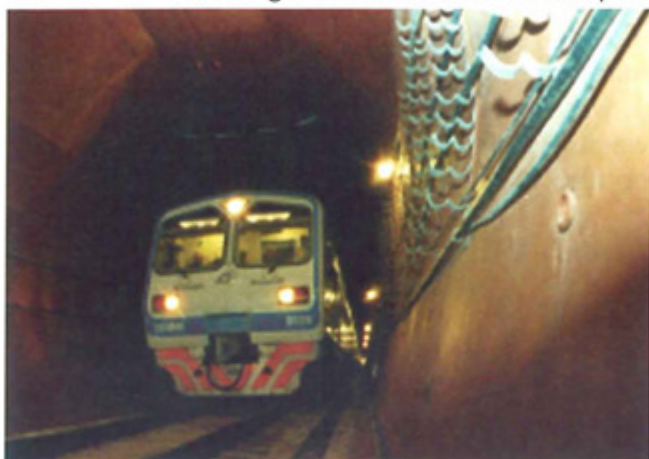
The tunnel view from the west Point
