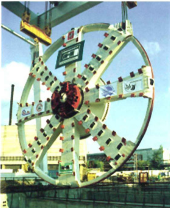
Cutting Head installation of the Herrenknecht shield
