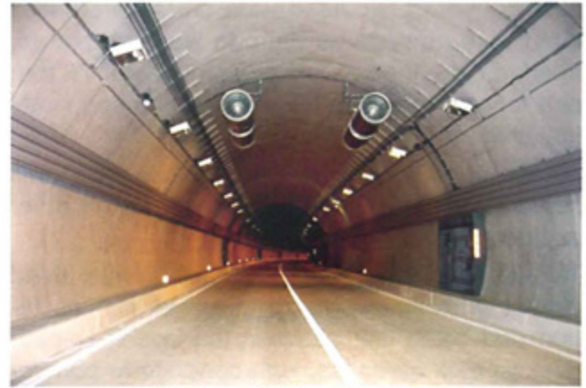
Inside view of Matssestinsky tunnel
