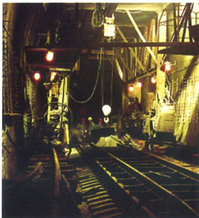
Permanent rail laying in the tunnel
