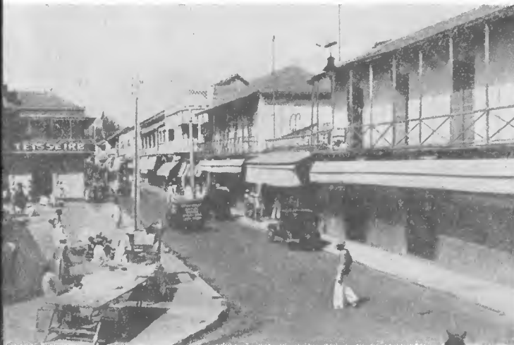
Rue des Essarts—near the market place.
