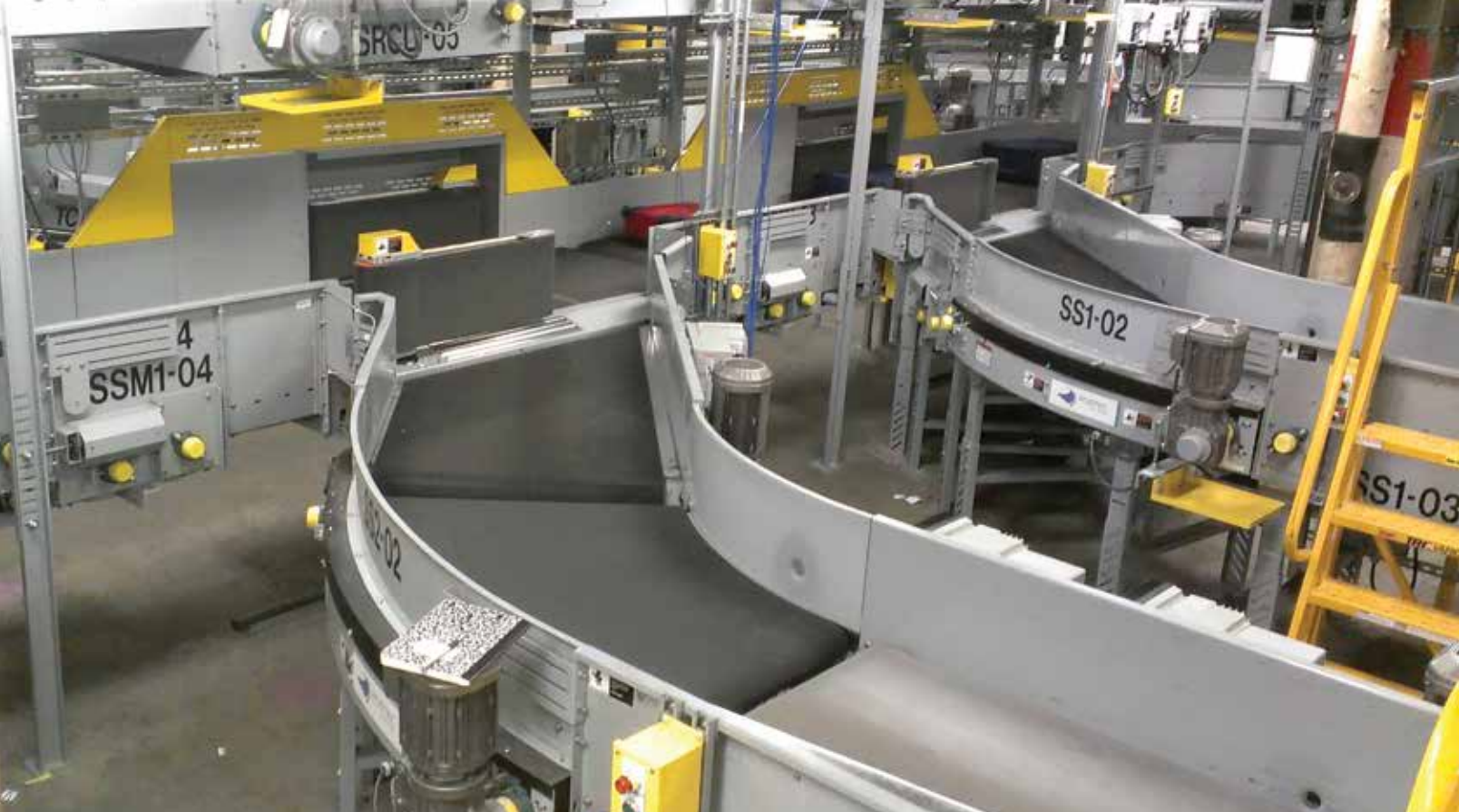
Fitting the new inline baggage system into an existing bag room instead of building a new facility saved an estimated $70 million.
