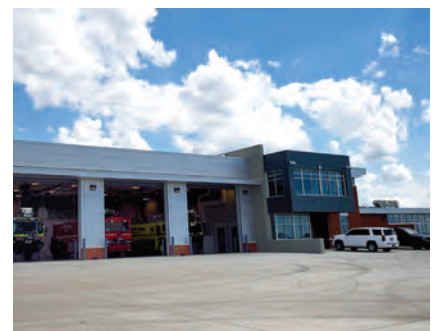
40 Lexington Blue Grass Airport Adds New Fire Station During Airfield Upgrades
