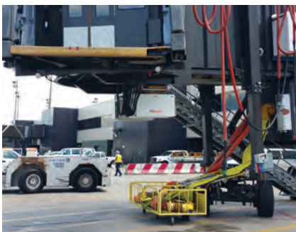
44 Ground Power Upgrades in the Works at Newark Int'l
