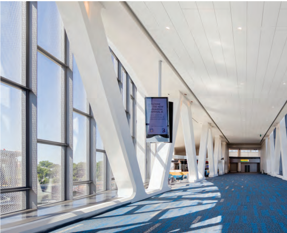
8 Pedestrian Bridge Facilitates Construction of New Arrivals & Departures Hall at LaGuardia Terminal B
