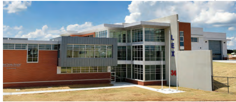
The new station includes lots of windows to provide crews as much natural light as possible.
