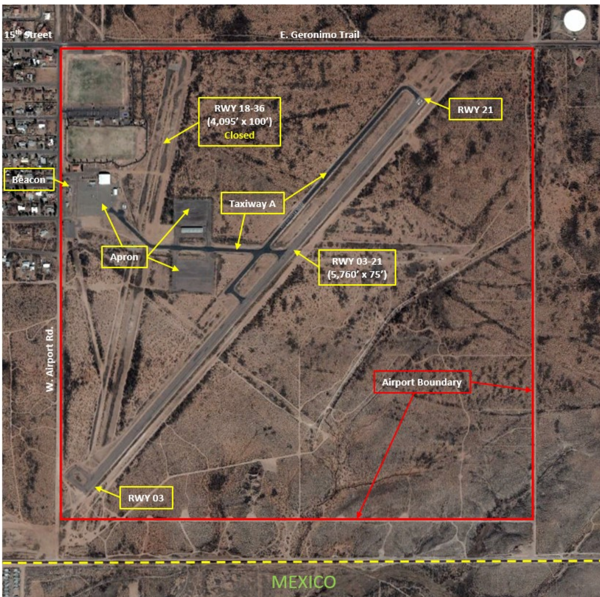
Exhibit 1-4. Current Airfield Facilities
