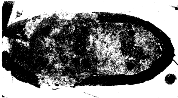
Fig. 18 – Severe corrosion condition on the aircraft aluminum skin where a discharger retainer was installed
