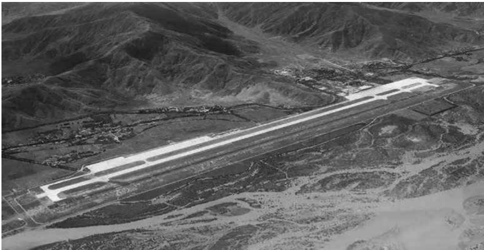
Fig 20: Chamdo Bangda Airport: Overview
