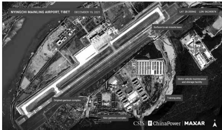
Fig 18: Nyingchi Airport: Overview
