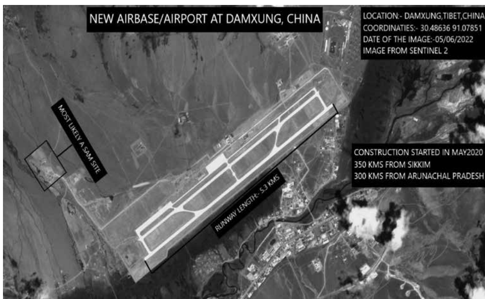
Fig 28: Infrastructure at Damxung Airport
