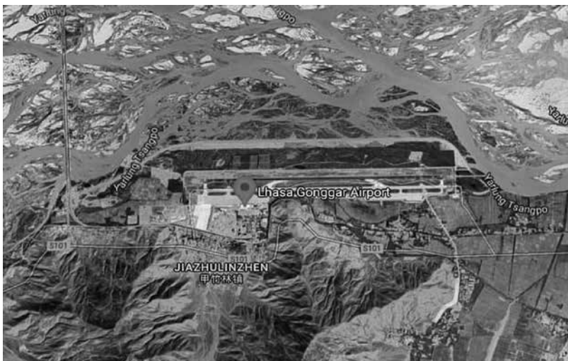
Fig 17: Lhasa Gonggar Airport: Overview
