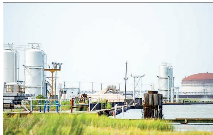
An LNG processing plant is seen in Cameron, Louisiana in August 2020. PHOTO: AFP/ ANDREW CABALLERO-REYNOLDS /FILE
