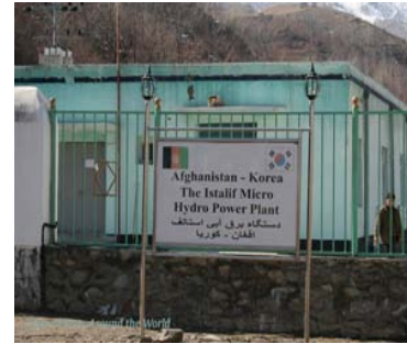
Istalif Power Plant, Power Plants around the World, 2010
