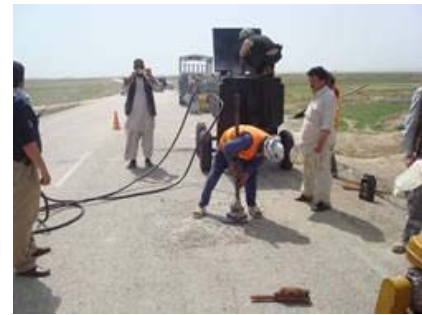
Afghan Road Maintenance Crew, AIRP, 2009
