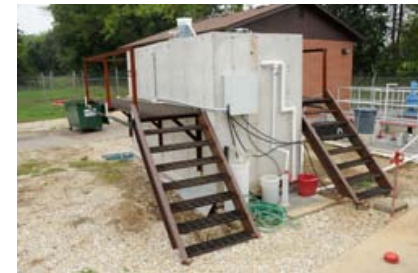
Wastewater Plant "In a Box" (Used with permission of the Missouri University of Science & Technology, 2009)
