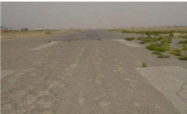
Kunduz Airport, Kunduz Province, Afghan Ministry of Transportation & Civil Aviation, 2010
