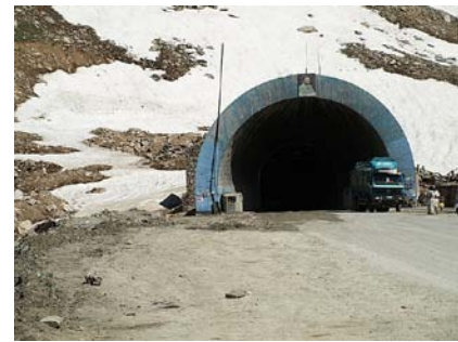
Salang Tunnel Entrance (Taken by Michael Vogt, Use under GNU Free Document License, Wikimedia Commons, June 2009)
