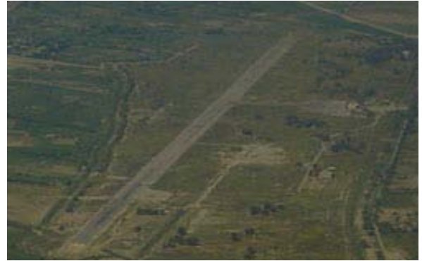
Jalalabad Airport, Nangarhar Province, Afghan Ministry of Transportation & Civil Aviation, 2010
