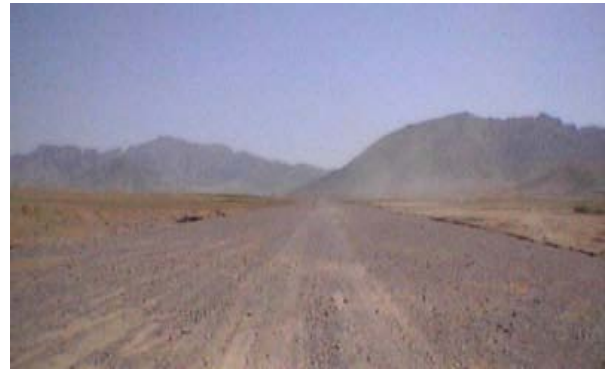
Rustag, Takhar Province, Afghan Ministry of Transportation & Civil Aviation, 2010
