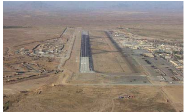
Kandahar International Airport, Kandahar Province, Afghan Ministry of Transportation & Civil Aviation, 2010
