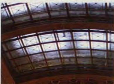
Below: Ceiling detail from the reading room
