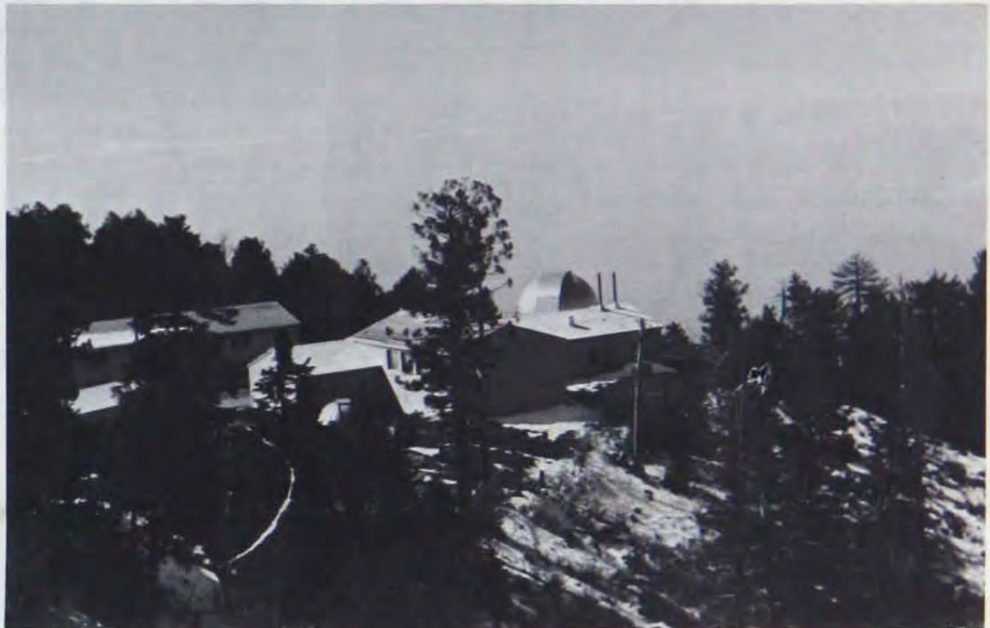
THE MT. LEMMON FACILITY is 17 miles northeast of Tucson, Arizona, and another 28 miles up the mountain. In addition to the observatory itself, the area has a laboratory-workroom building, living quarters and a gymnasium.
