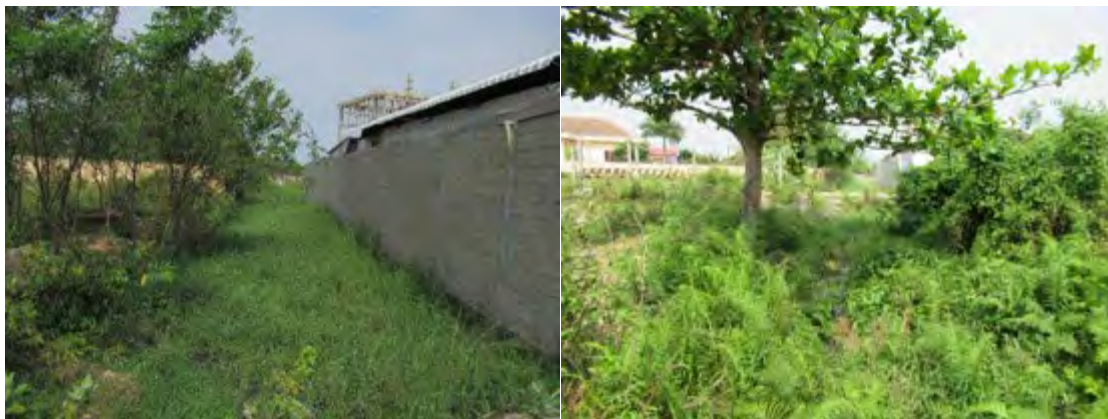
Condition of drainage canal
