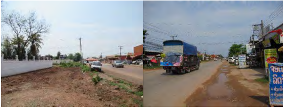
Condition of the drainage near crossing drainage on road 13N
