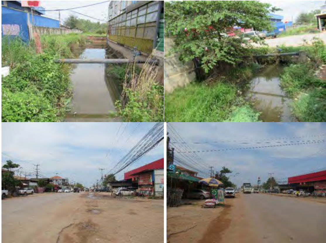
Condition of crossing drainage.
