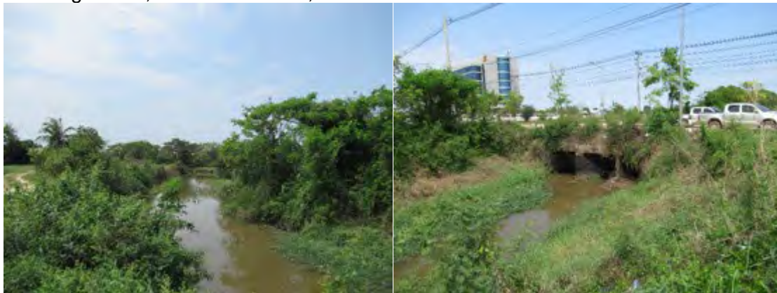
Condition of the drainage canal.
