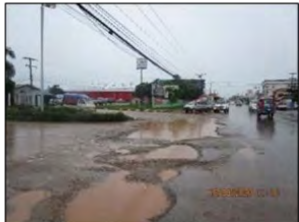
No existing ditch (pavement edges are severely deteriorated)
