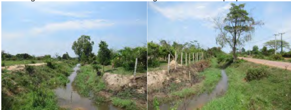
Condition of the drainage canal
