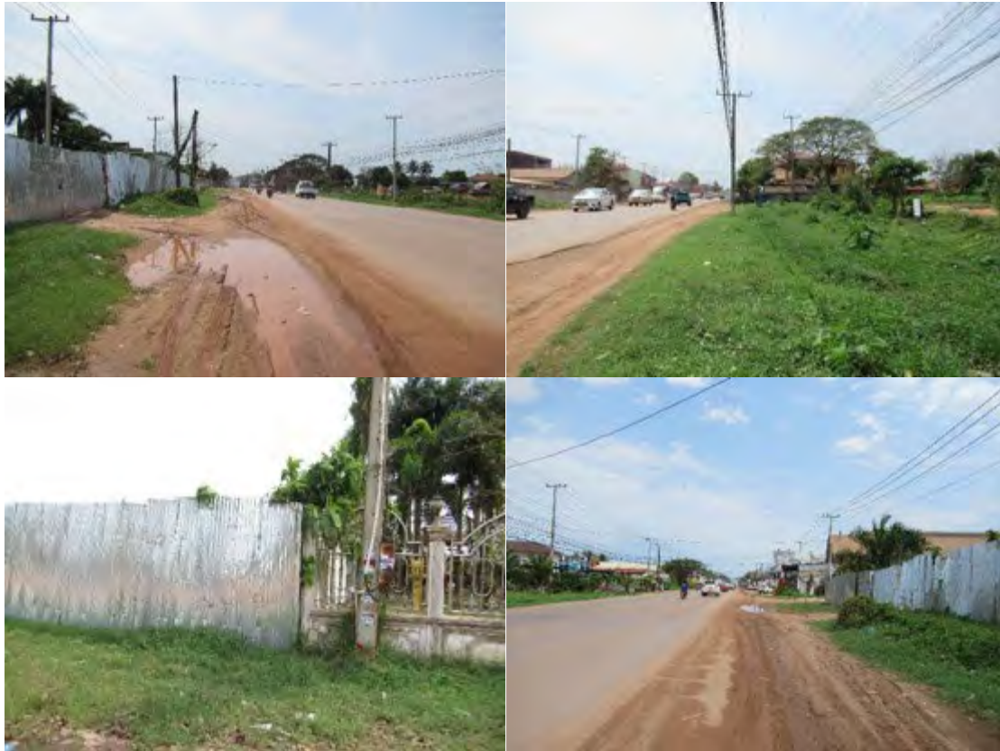
Condition of road sides where the canal no. 4 will pass
