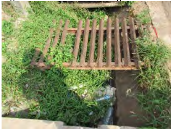
Existing road side drainage condition
