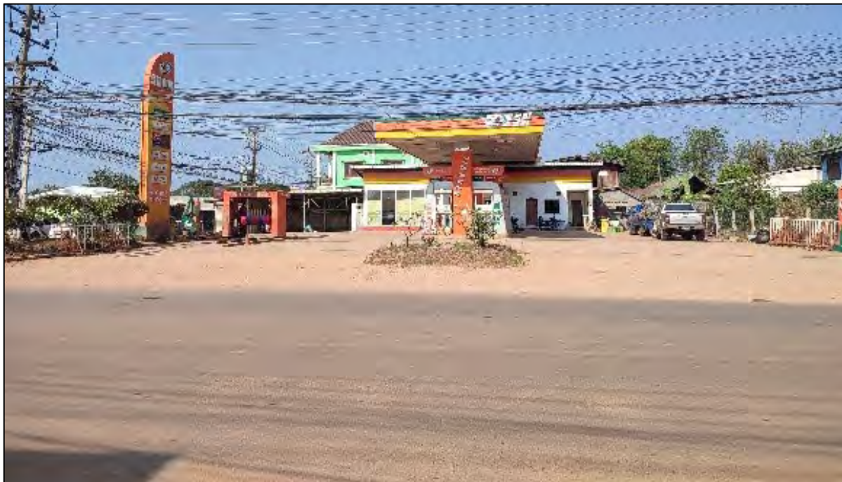
Figure 17: Gas Station 03 (KM11.1)
