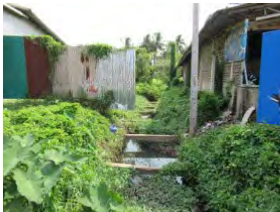
Crossing drainage on Road 13N
