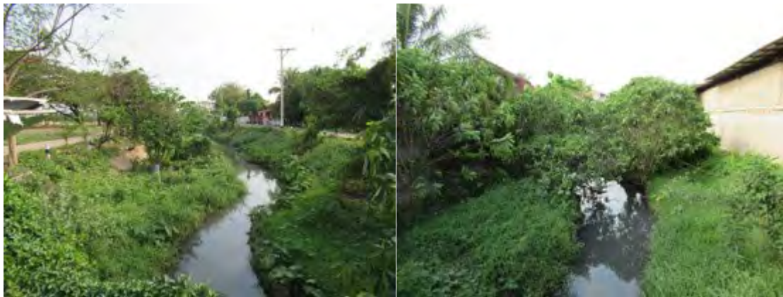
Condition of drainage in Ban Dongnasok area
