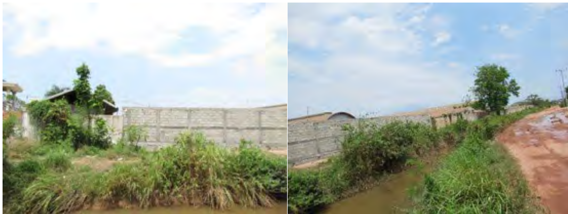
Condition of the drainage canal
