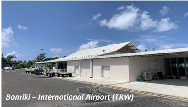
Figure 5 Bonriki Airport at Completion
