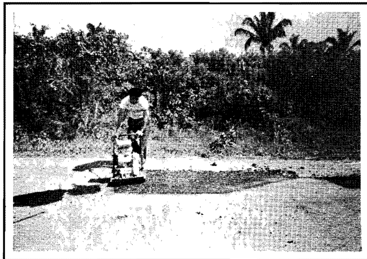
COMPACTING THE PATCH
