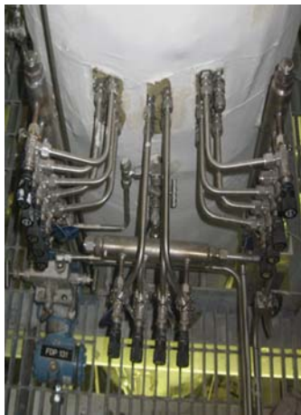
FIGURE 36: Photo of variable-position throttle valve located at the entrance of each helical coil.
