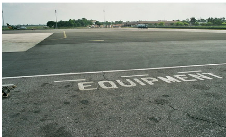
Photo 1: Rehabilitation of the Runway at JNIA
