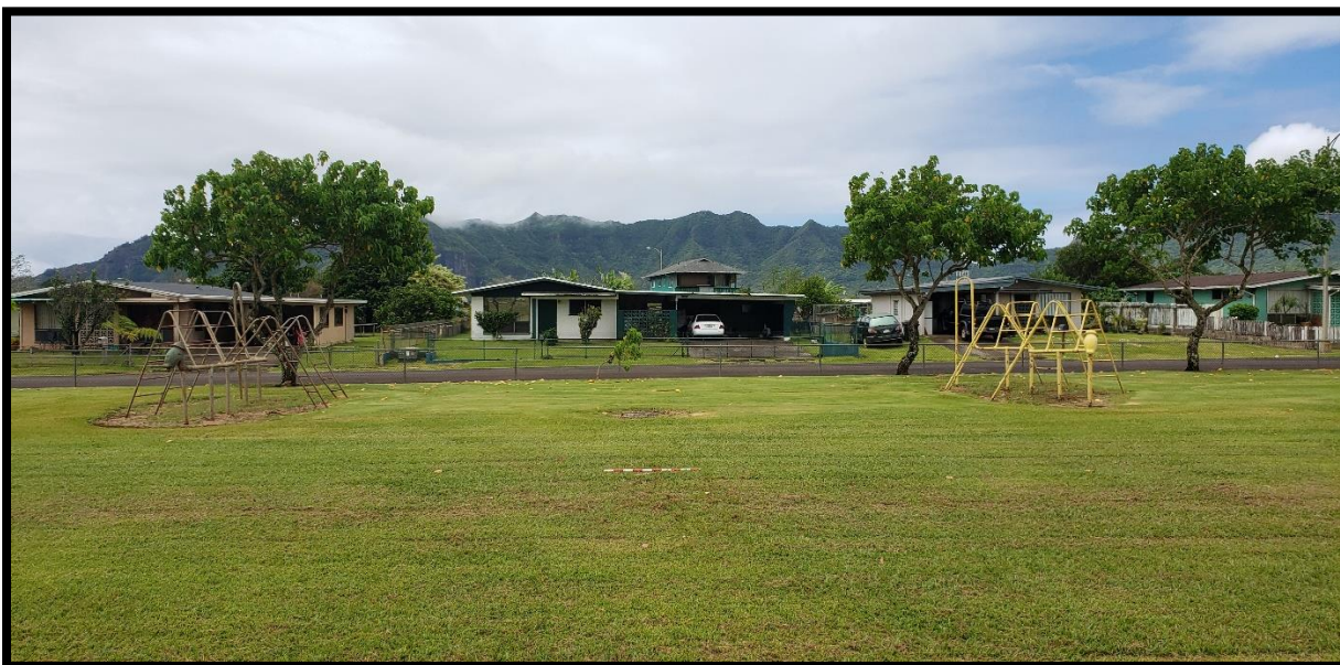
Figure 22. Overview photo of play structures and small concrete slab located in the middle of the project area looking south
