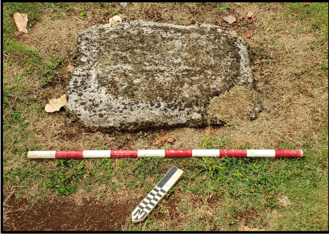
Figure 25. Close-up photo showing small concrete slab present between the two play structures
