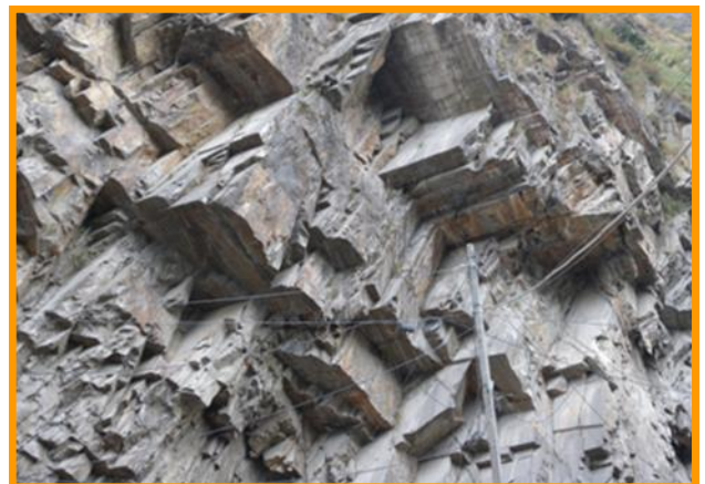
Figure 1. Confronted with this potentially unstable jointed rock slope, multiple reasons for the overbreak and instability suggest themselves. There are clearly adverse values of JRC, JCS, and \phi_r , and there are also adverse ratings of Jn, Jr, Ja (and Jw on occasion).
