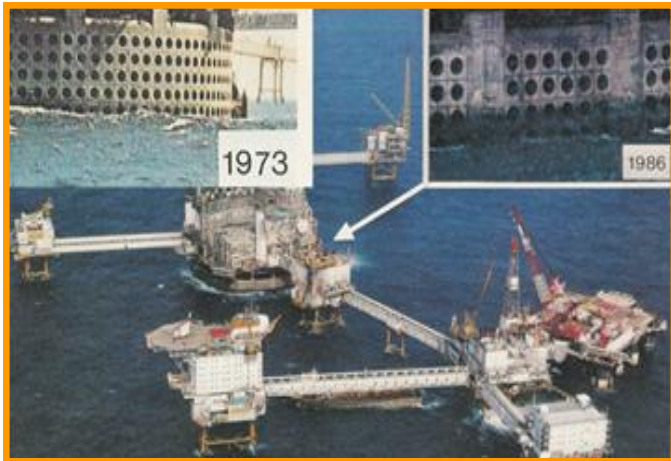
Figure 9. A view of the Ekofisk reservoir in the North Sea, where compaction of the jointed-chalk reservoir of 300 m thickness at 3 km depth caused increasing sea-bed subsidence that amounted to about 4 m when investigations began in 1985-1987. Now it is 10m.
