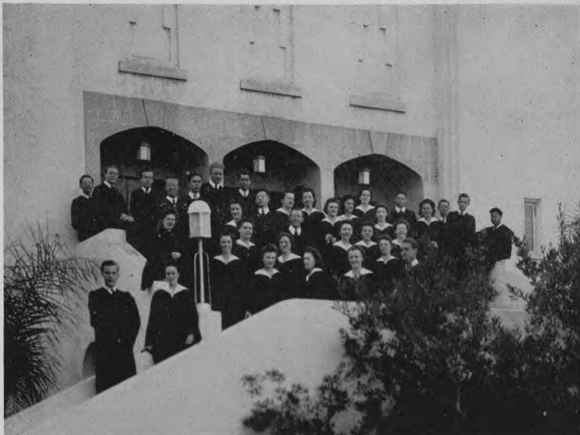
Coming Down Hole Memorial Auditorium Steps
