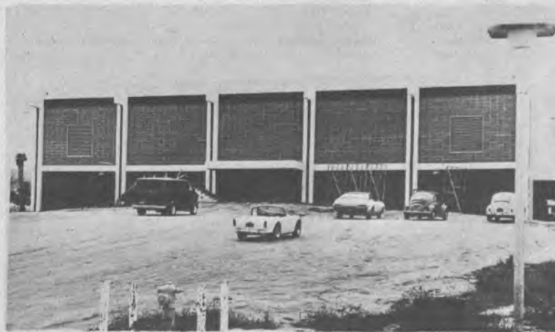
The bare dirt slope behind the gym. Work to transform this eroded bank will begin soon.
