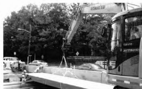
A New Jersey bridge takes shape with the hybrid-composite beam
