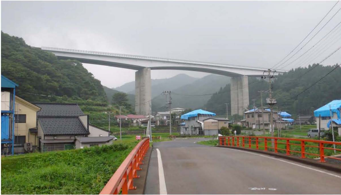
Fig. 6.5. Omigawa Bridges on the Horukiru Expressway.
