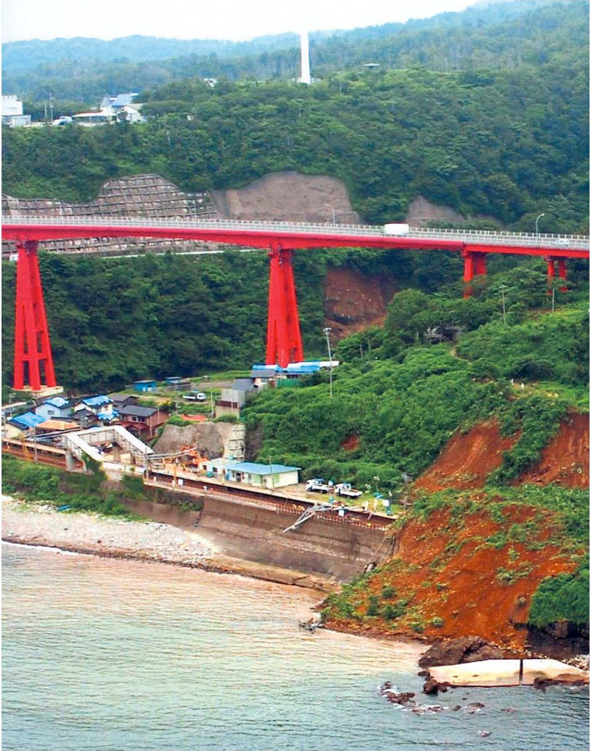
Fig. 6.21. Yoneyama Bridge and landslide.
