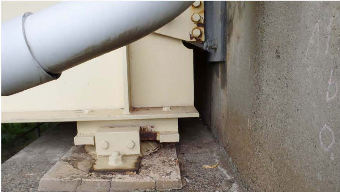
Fig. 6.9. Bearing at south abutment of Yoshiigawa Bridges.
