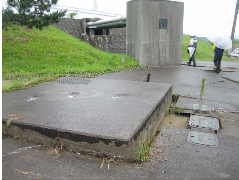
Figure 4.4: Kai-Un Bridge over Sabaishi River (Site N37.39233°, E138.58063°, 7/19/2007, 1:40 p.m.). A water cistern near the pipeline rupture uplifted in liquefied ground.
