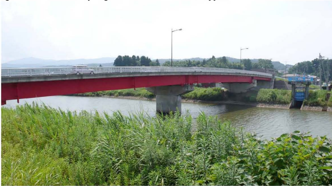
Fig. 6.65 View looking south across the Ugawa River at this steel bridge.
