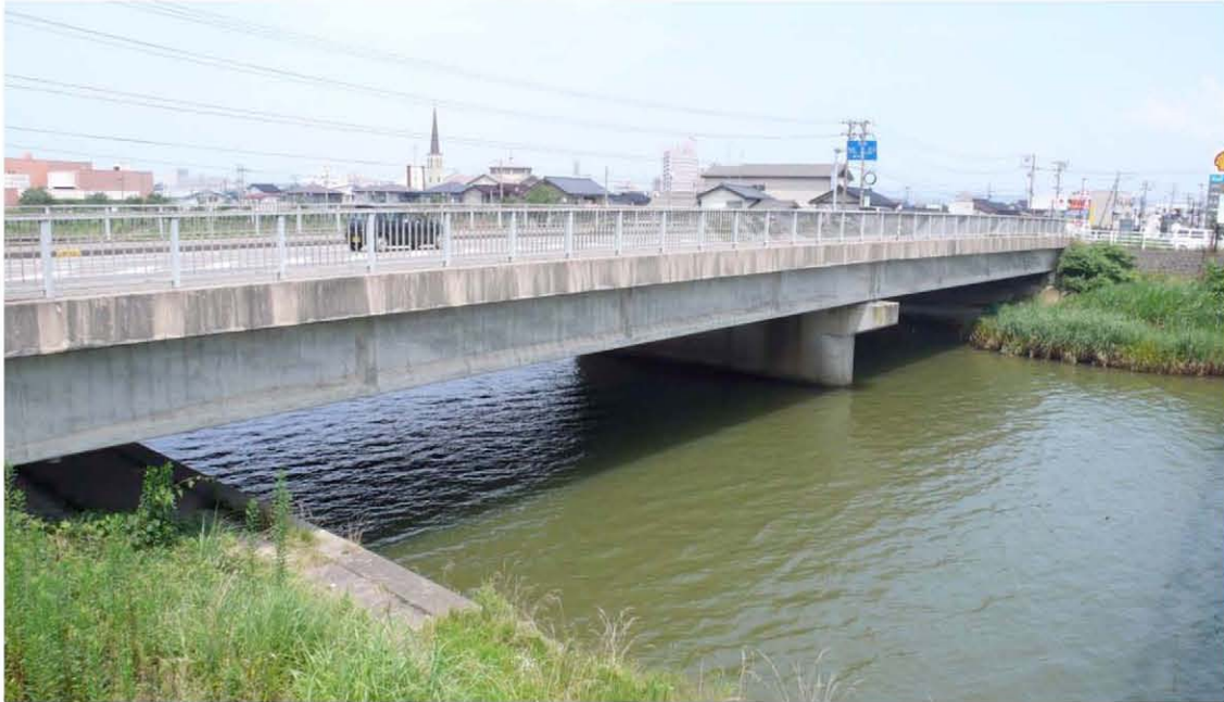
Fig. 6.18. Highway 80 Bridge across the Ugawa.
