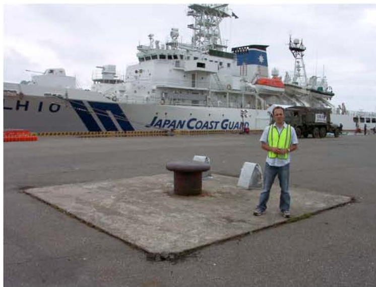
Photo 8.24: Kashiwazaki Port - Evidence of minor settlement adjacent to a pile-supported (?) bollard anchorage located along the northern face of the terminal used as the berth for the Japan Coast Guard (Site SD8, N37.36680° E138.53825°, photo taken 7/22/07 15:21).
