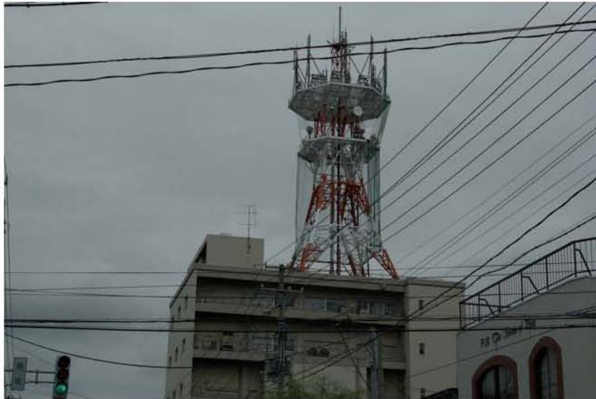
Figure 10.8: NTT communications building in downtown Kashiwazaki (Site SD20, N37.36847° E138.55813°, photo taken 7/23/07). No evidence of major structural damage to the tower was observed however no information on the performance of the electronics was available at the time of the investigation.
