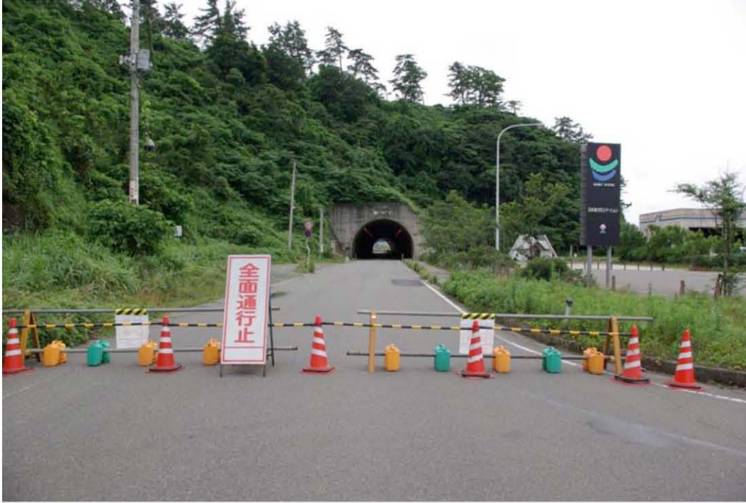
Figure 9.8: Tunnel was initially open to traffic following earthquake, but subsequently closed as of July 22 nd (Site SD4, N37.38439° E138.60083°, photo taken 7/22/07 13:36). Damage to tunnel was not observed, but landsliding and toppled monuments on top of the tunnel was observed.
