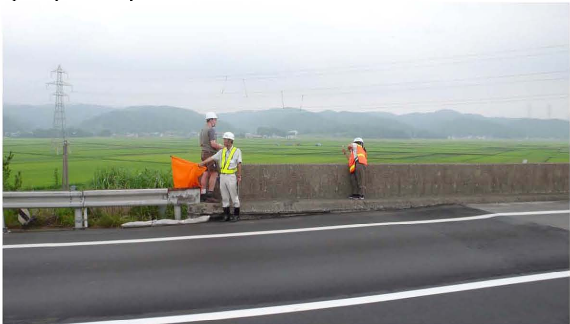
Fig. 6.10 Repaired embankment and approach slab at Yoshiigawa Bridges.
