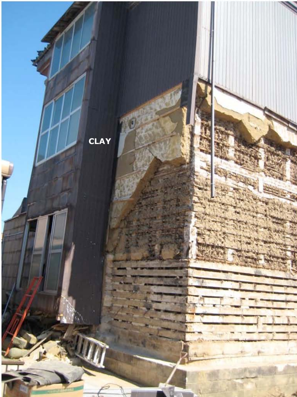
Figure 5.11: Traditional Japanese tsumi-kabe (“soil wall”) construction technique (Site SP13, N37.37056°, E138.55694°).
