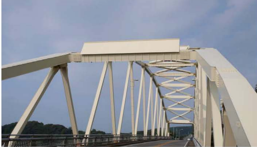
Fig. 6.24. Looking at the struts and cross-bracing of the Yonahime Bridge.
