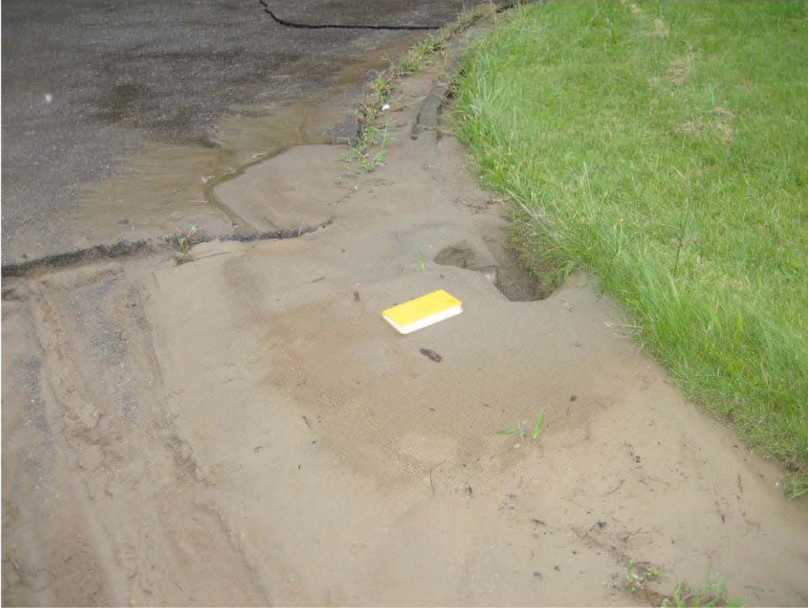
Figure 4.17: Kashiwazaki Wastewater Treatment Plant on the south side of Sabaishi River near its outlet to the Sea of Japan (Site RK9 N37.38748° E138.56587°, 7/19/2007). Liquefaction features were abundant near the wastewater treatment facility.
