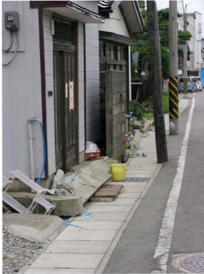
Fig. 4.42: Downtown Kashiwazaki Lateral Spread (SiteYT24, N37.36963°, E138.5486°, photo taken 7/22/07, SiteYT24_YT_03 as shown in Fig. 4.40).
