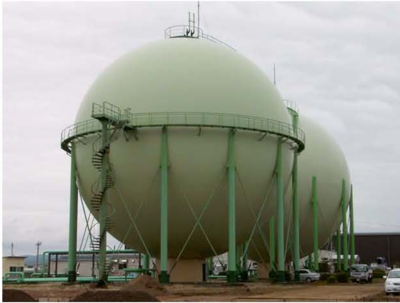
Figure 7.10: Steel natural gas tanks undergoing inspection by the operator and engineering consultants (Site SD13/RK57, N37.37253°, E138.59488°, photo taken 7/23/07 12:37). Trenching and below grade inspections had already taken place prior to the field investigation. No damage was observed to the tanks, pipe connections, or mains, however observations were made from the perimeter of the facility, a short distance from the structures.
