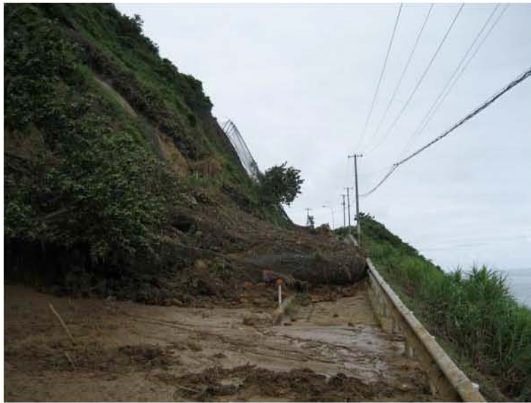
Figure 3.2: Coastal landslides on Highway 352 north of Kashiwazaki-Kariwa Nuclear Power Plant at road closure south of Route 373 (Site RK34; N37.48455° E138.62435°, photos taken 7/22/07 at approx. 10:45). This area consisted of at least eight individual slides. The landslide shown in the bottom photo consists of a slide in an area of previous instability - a shotcrete stabilization system is in effect for the bottom 50 m of this slope (total slope height is ~115 m), and overlain with a wire-mesh rock deflection system. The slide is approximately 50 to 60 m wide, 65 m long, and less than 1 meter thick. The landslide initiated above the shotcrete slope, moved into the wire-mesh and caused failure of the meshing and pull-out of the steel supports. The wire-mesh restrained most of debris, depositing the majority on the road, with only a slight quantity of the debris sliding over the road edge. The failure plane inclination is approximately 60°.
