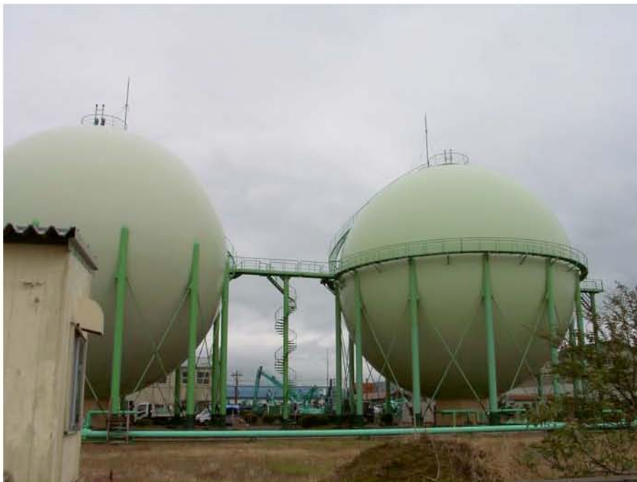
Figure 7.11: Steel natural gas tanks undergoing inspection by the operator and engineering consultants (Site SD13/RK57, N37.37253° E138.59488°, photo taken 7/23/07 12:31).
