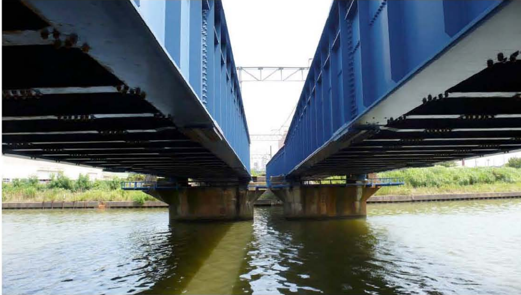
Fig. 6.63. Looking under the Railway Bridges.
