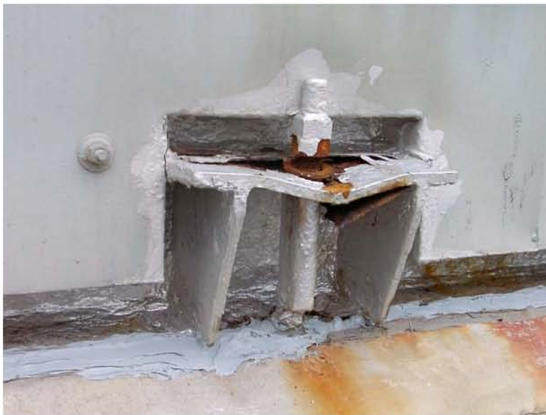
Figure 7.6: Kashiwazaki Port - Anchorage of asphalt storage tank (Located near Site RK25, N37.36713° E138.53210°, photo taken 7/22/07 12:37).
