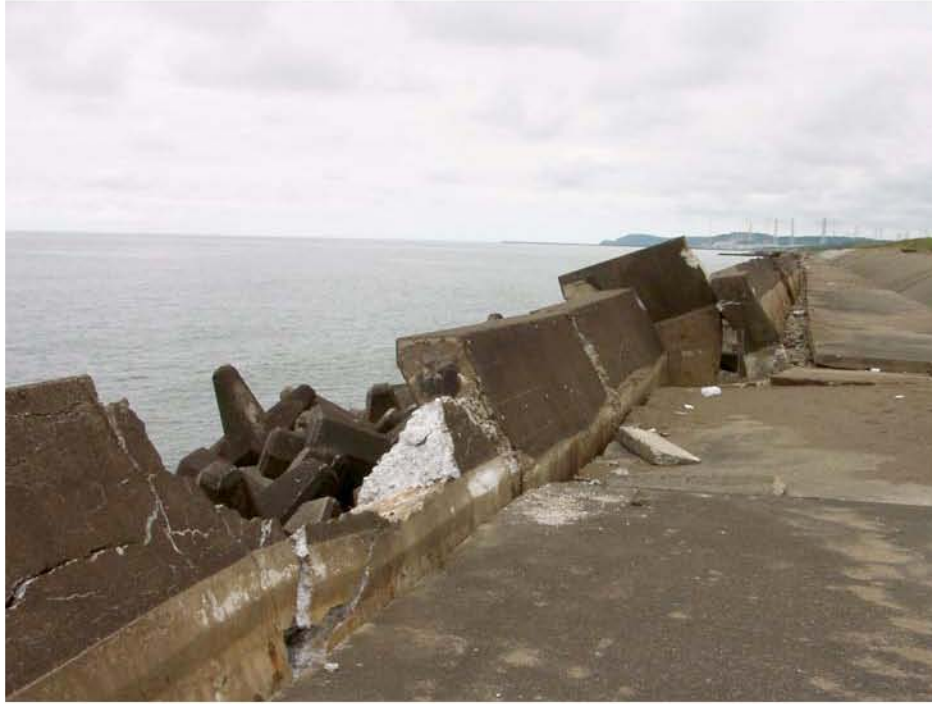
Figure 8.39: Lateral displacement, rotation, and structural damage to the seawall (Location is southwest of Site SD1, photo taken 7/22/07 11:45).
