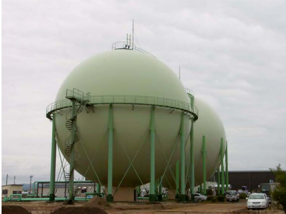
Figure 10.11: Natural gas tanks being inspected by local engineers (Site SD13/RK57, N37.37253° E138.59488°, photo taken 7/23/07). Very minor ground settlement and later movement near ditches was observed in the vicinity but the no damage was apparent to the tank foundations, appurtenant piping, or the tanks.
