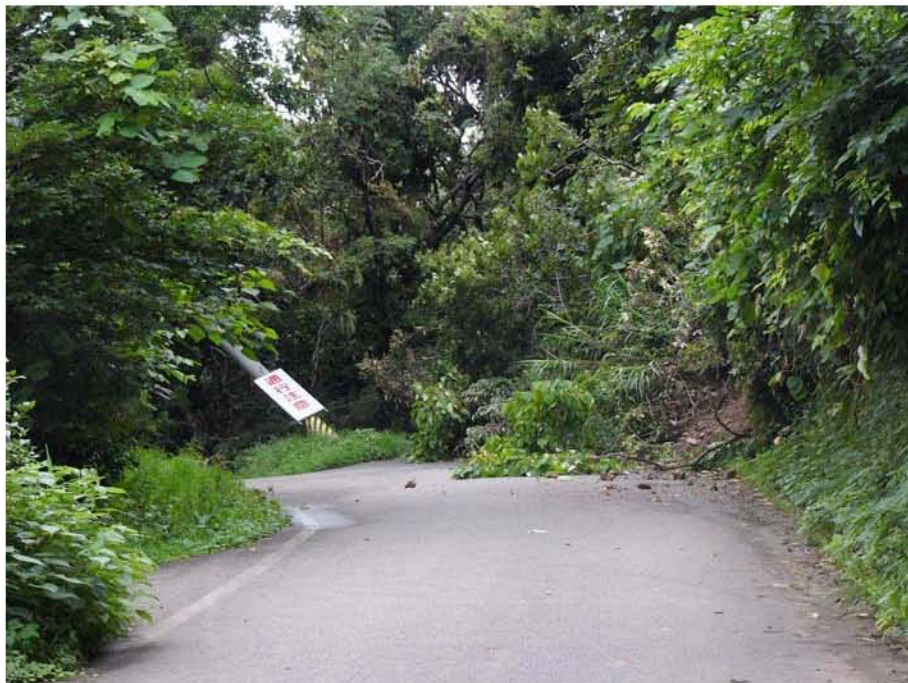
Figure 3.4: Yoneyama Landslide, located south of Kashiwazaki (Site YT17; N37.32223° E138.43828°, photos taken 7/21/07 at approximately 15:20). This slide marked the southwest-most limit of observed landslides along the Sea of Japan coast. The slide extended to the full height of the slope and blocked a paved coastal access road.
