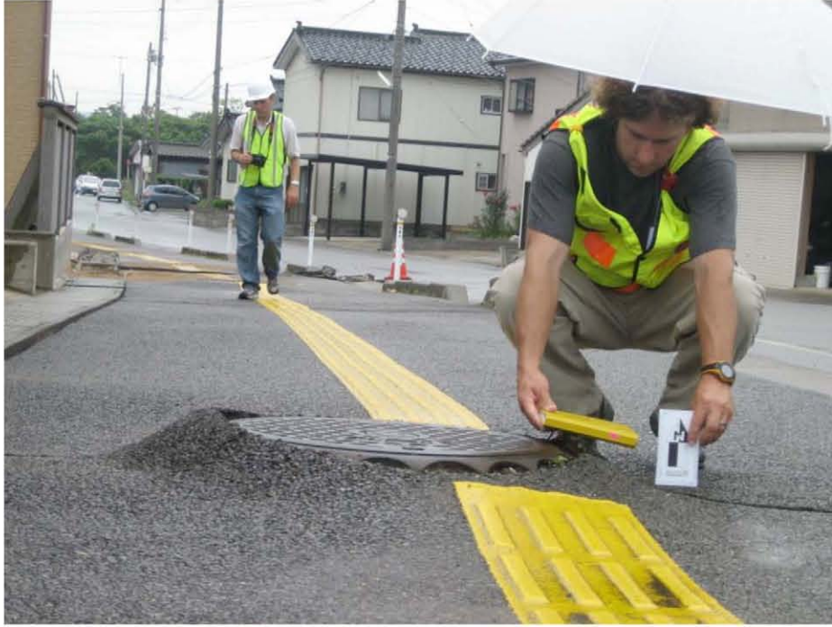
Figure 4.6: Kai-Un Bridge area Sabaishi River (Site RK4 N37.39233° E138.58063°, 7/19/2007, 1:40 p.m.). Numerous manholes on the southeast bank near the Sabaishi River uplifted in liquefied ground.
