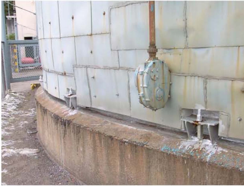
Figure 8.9: Kashiwazaki Port - Anchorage of asphalt storage tank (Located near Site RK25, N37.36713° E138.53210°, photo taken 7/22/07 12:37).
