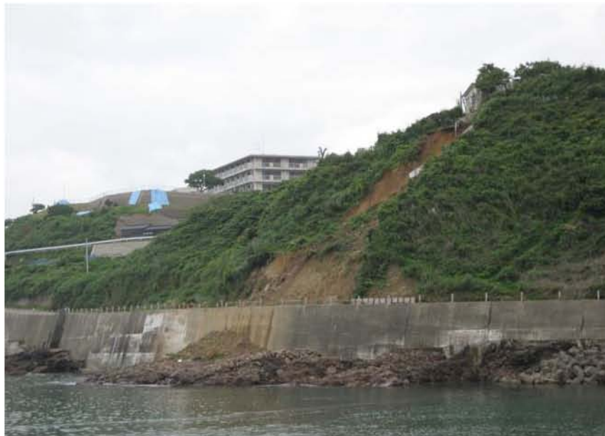
Figure 3.1: Shallow colluvial landslide located just north of the Kasashima Fishing Village, Site RK22/SA10; N37.33802° E138.46995°, photos taken 7/20/07 15:57 (top) and 7/21/07 13:35 (bottom). Dimensions are approximately 36 m wide, 24 m tall, 2 m thick. The lithology is composed of 24 m of weak mudstone overlying 6 m of more indurated, brecciated mudstone, which outcrops at the road. A 10 m tall concrete seawall leads down to the brecciated mudstone shore platform. The slide occurred in weak mudstone/colluvium, sliding over the brecciated mudstone, onto the road, and over the edge of the concrete seawall, spilling debris onto the shore platform at ocean's edge.
