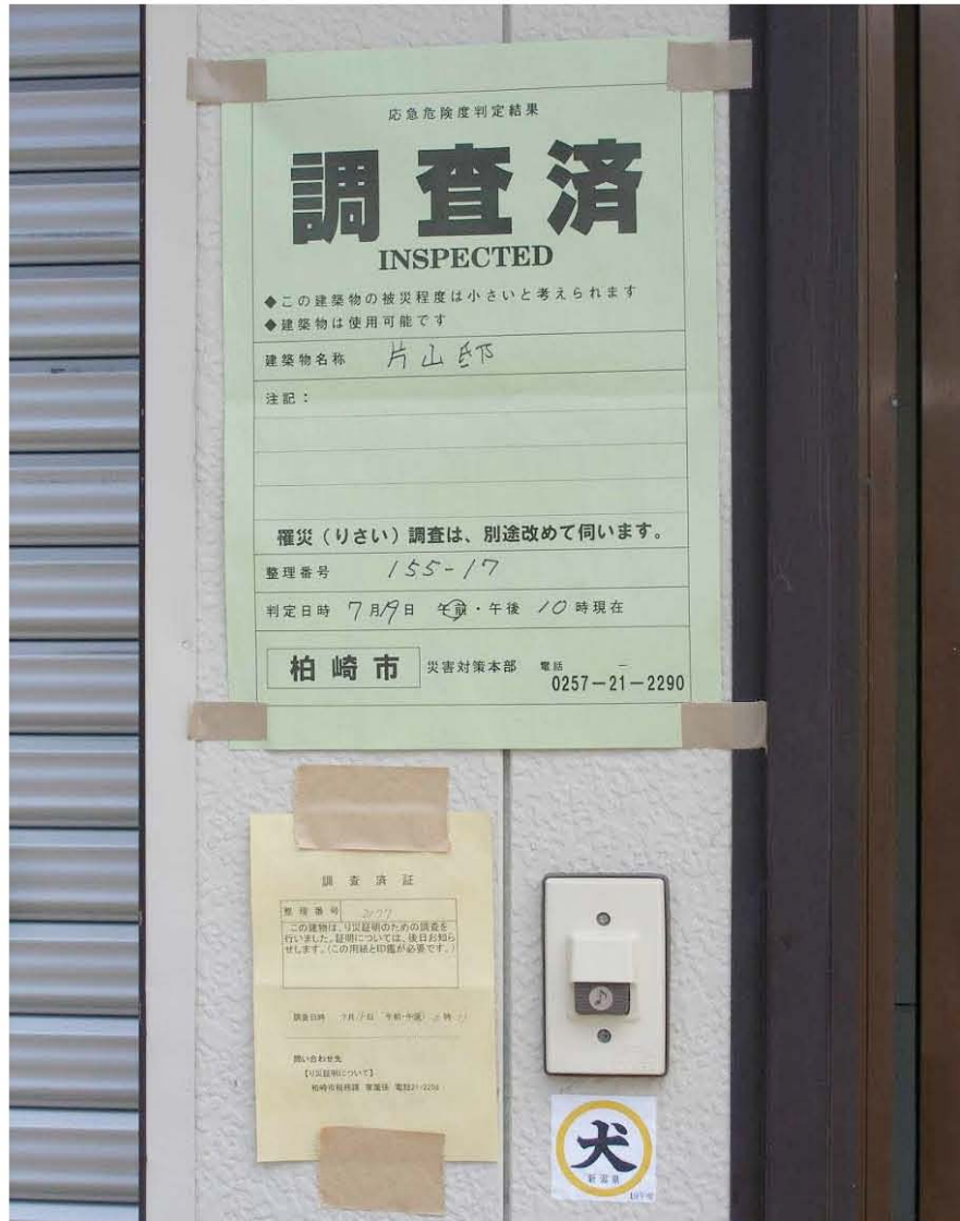
Figure 11.7: A building in Kashiwazaki city that has been through two surveys, with both a green tag as well as a standard yellow notice that the damage certification survey has also been completed.
