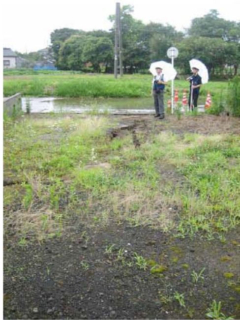
Figure 4.8: Kai-Un Bridge area Sabaishi River (Site RK4 N37.39233° E138.58063°, 7/19/2007, 1:40 p.m.). A sub-linear zone of lateral spreading, sand boils and settlement that may be associated with a buried shoestring sand deposit from the former channel of the Sabaishi River resulted in damage in the neighborhood immediately south of the Kai-Un Bridge.
