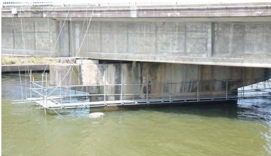
Fig. 6.54. Pier supporting Rinko Yasaka Bridge.
