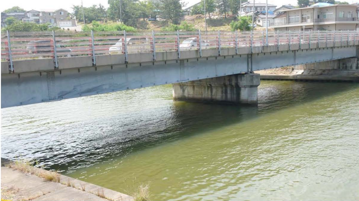
Fig. 6.55. The Yasaka Bridge.
