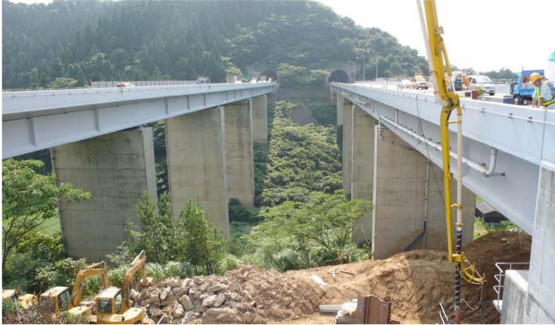
Fig. 6.2. Looking south at the Hachisaki Bridges.
