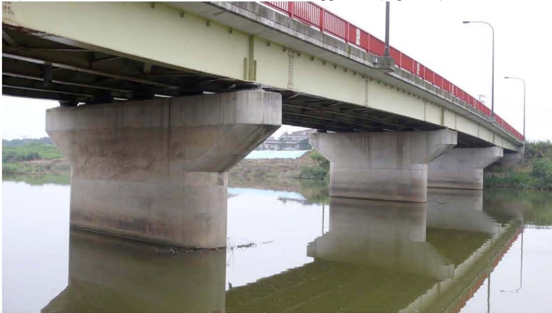
Fig. 6.40. The four, steel 'I' girder span Kaiun Bridge on pier walls and seat abutments.
