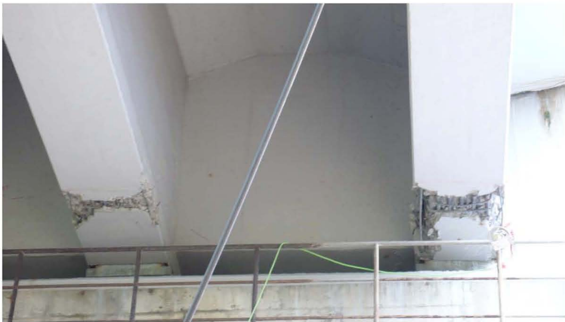
Fig. 6.4. Closer view of girders on the west Hachisaki Bridge.
