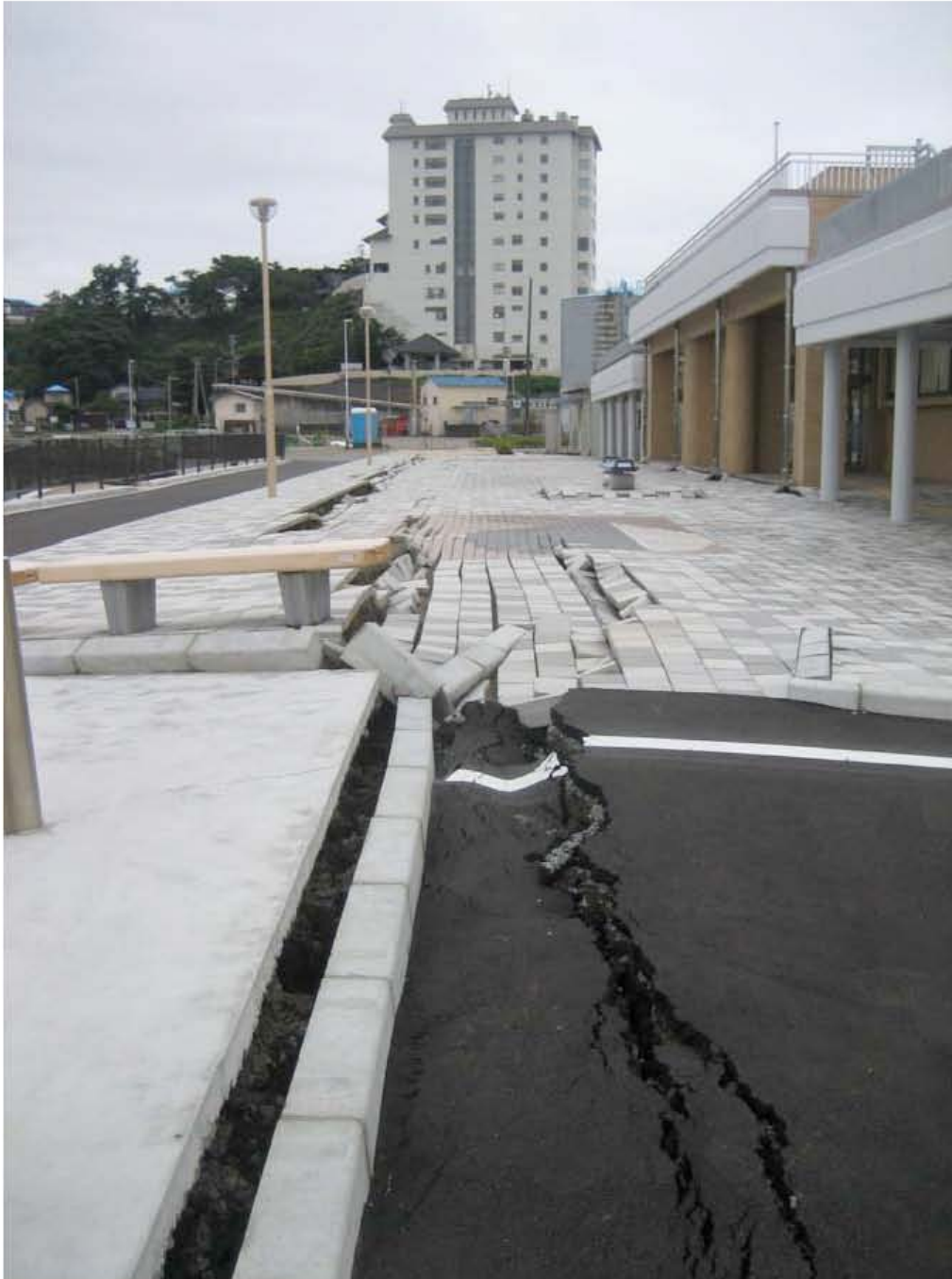
Figure 4.21: Kashiwazaki Harbor - The southern area experienced ground damage from liquefaction-induced lateral spreading and settlement. A harbor-front caisson rotated toward the harbor, to the left of the photo, initiating lateral displacement of the soil behind it, between the caisson and port building (Site RK25, N37.36713° E138.53210°, 7/20/2007).
