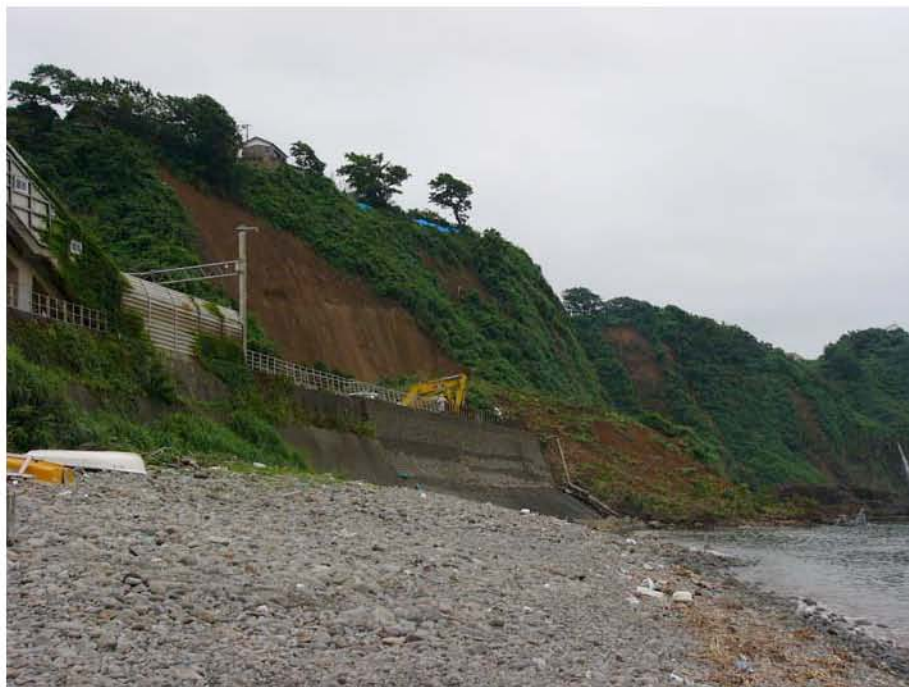
Figure 3.5: Landslide at the Oumigawa Train Station on the Shin-etsu Line (Site RK20/SA9/YT16; N37.34200° E138.48888°, photos taken 7/21/07 12:48 (top) and 7/24/07 15:00 (bottom)). This was among the largest of the coastal landslides to the south of Kashiwazaki. Site access was not possible due to construction repairs. Note that slope stability in this area has been a problem, as seen by the railway tunnel protection structure immediately behind (to the south) of this landslide. Many more smaller landslides were observed to the north and south of this location.
