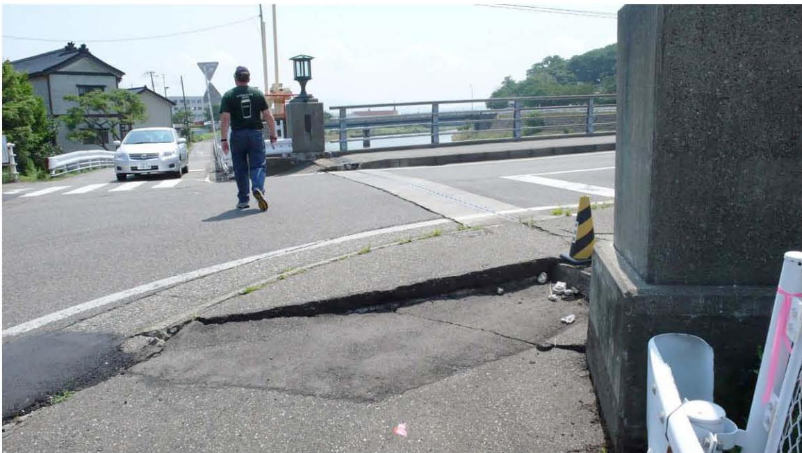
Fig. 6.58. Approach to Ukawa Bridge.
