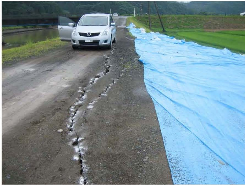
Figure 4.1: Fujii Weir downstream from Tashiou Bridge crossing of river. (Site RK16; N 37.34875^{\circ} E 138.61670^{\circ} , visited 7/21/2007 11:28 am UTZ+8). Extensive cracking of levee embankment.
