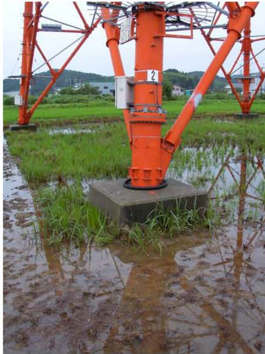
Figure 10.7: High voltage power line towers located in an area of soft ground (Site RK12, N37.44113° E138.63390°, photo taken 7/21/07). No evidence of ground failure, settlement, or structural damage to the towers was observed.
