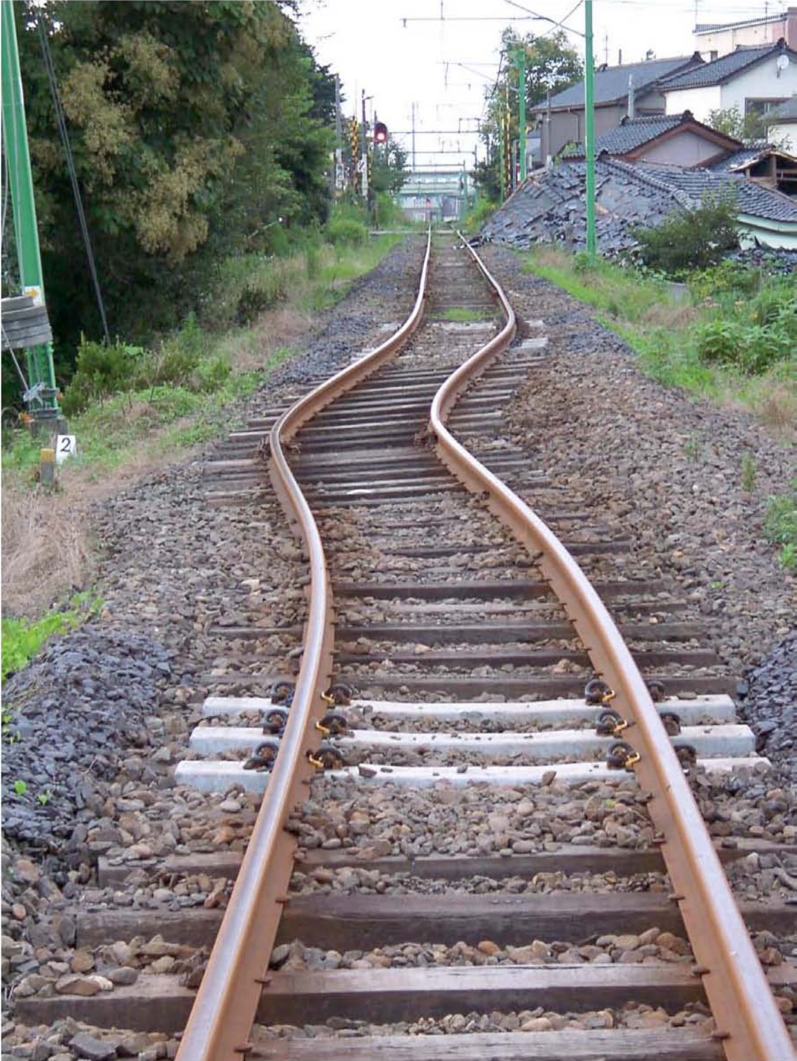
Figure 9.13: Lateral railway buckling (Site RK28, N37.37037° E138.56475°, 7/21/07 18:01).
