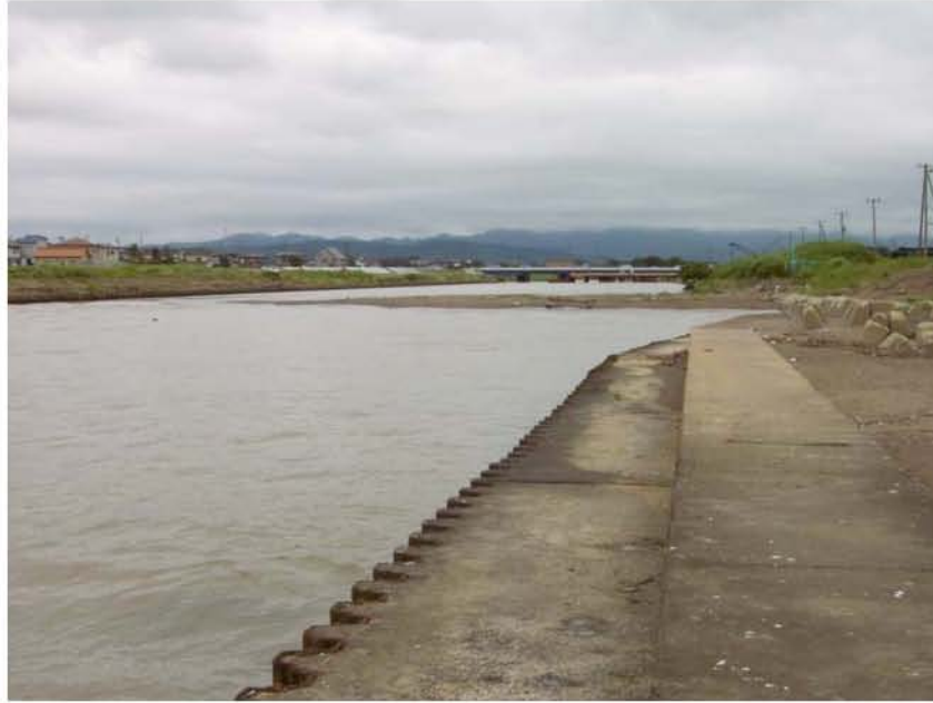
Figure 8.31: Mouth of the Sabaishi River showing the erosion control measures (Site SD 1, approximately N37.38868° E138.56508°, photo taken 7/22/07 11:07). The Ansei Bridge (Sites SA6/SD2/RK8) is visible in the background.
