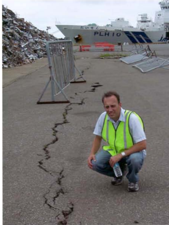
Figure 8.22: Kashiwazaki Port - Minor ground cracks located parallel to the western quay wall used as the berth for the Japan Coast Guard (Site SD8, N37.36680° E138.53825°, photo taken 7/22/07 15:17).
