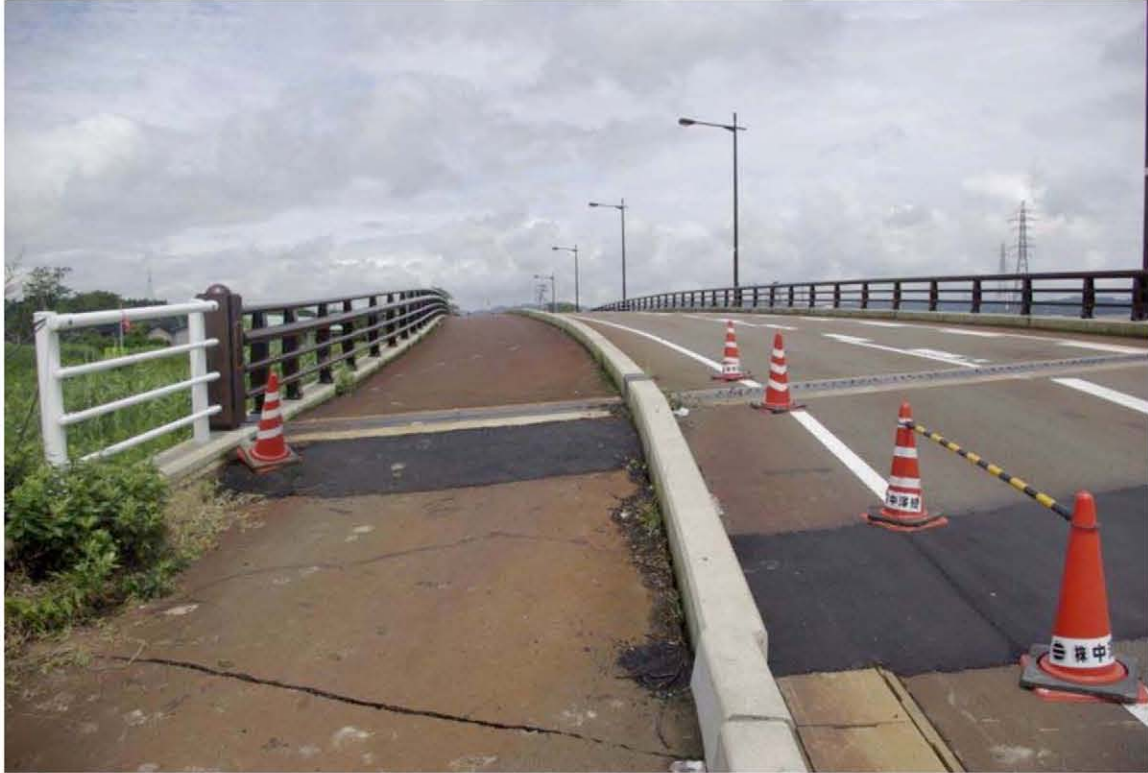
Fig 47. Repairs to bridge approach on Nagomi Bridge (photo courtesy of Scott Brandenburg).
