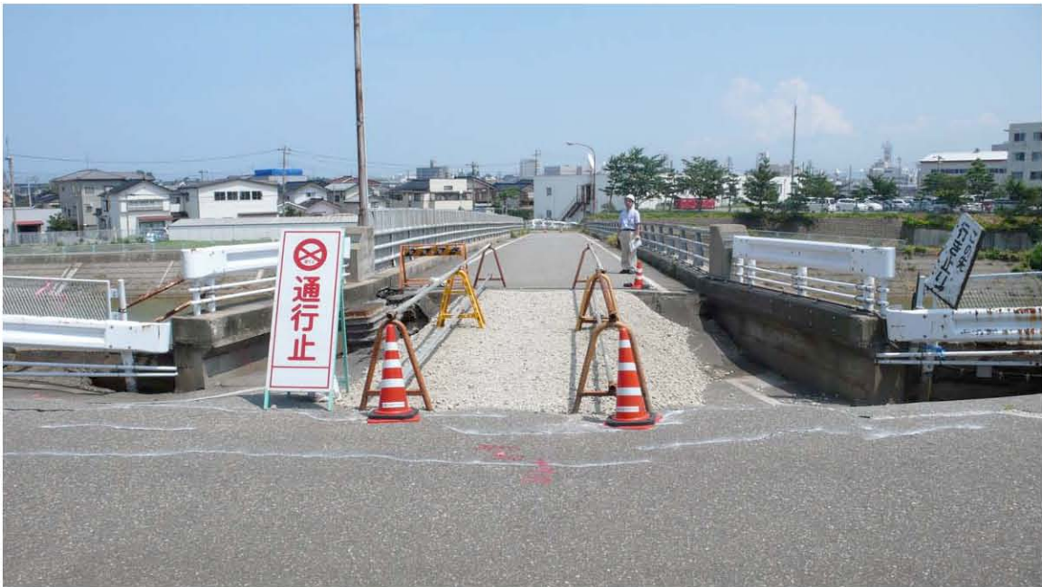
Fig. 6.60. Looking north at the south approach to Osu Bashi.
