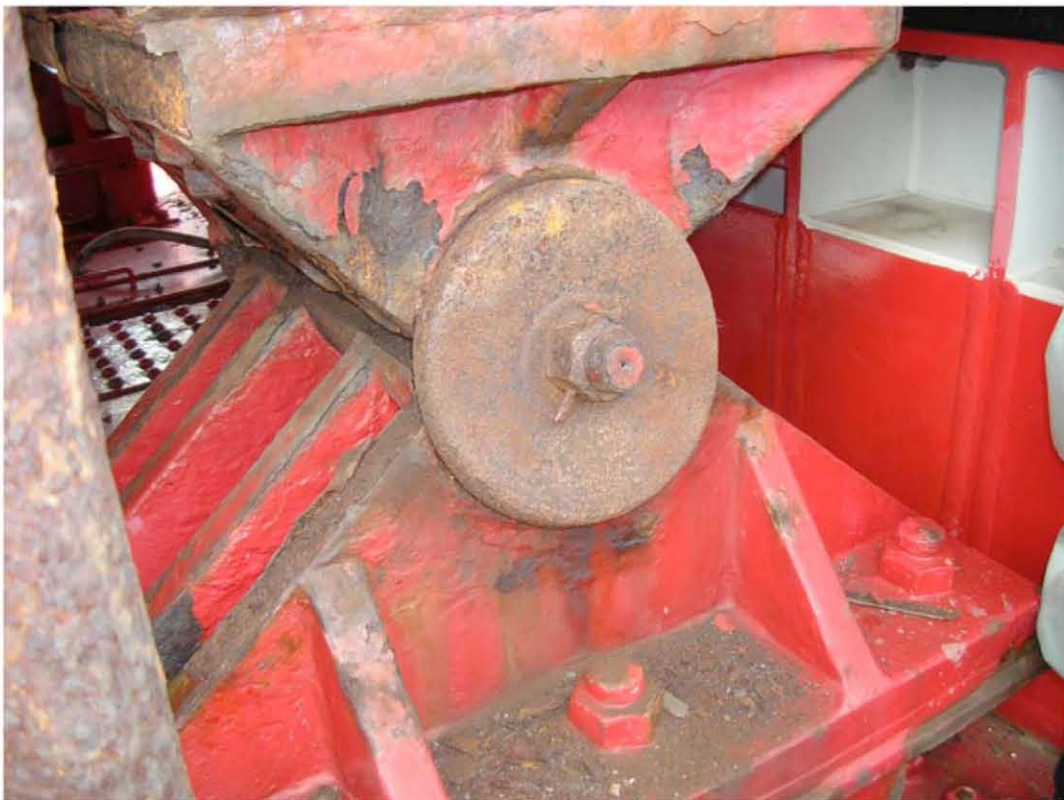
Fig. 6.23. Deformation of Bearing Pin-Cap caused by uplift force (courtesy of S. Unjoh, PWRI).
