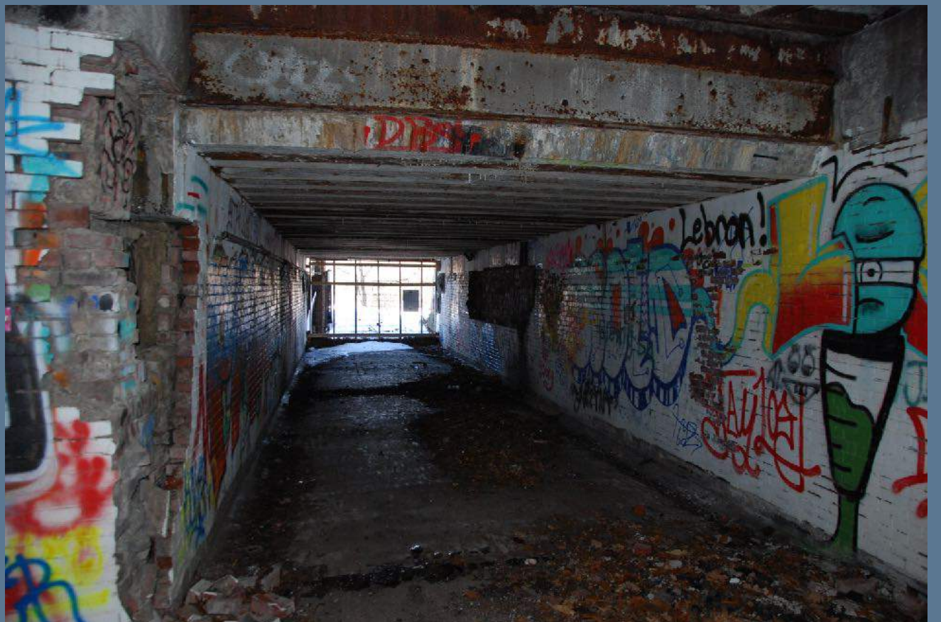
Train Depot - demolished
