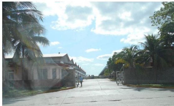
Logistics Facilities of Zelcom
