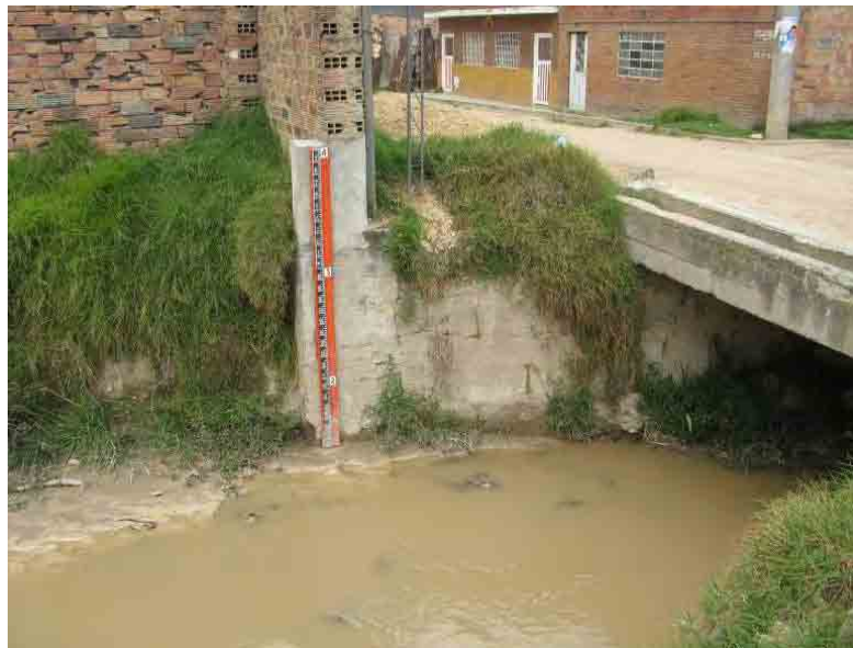
Photo S6-2-6 Photo of Llano Grande Section
