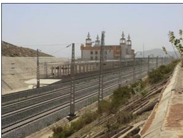
Adama Station and Double Track (Sebeta – Adama) Source: JICA Survey Team
