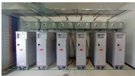
Photo 3.15 :Airfield Lighting CCR Unit
