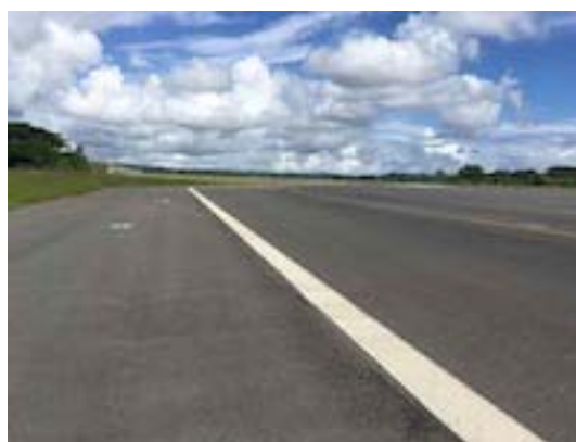
Photo 3.2 Turning Pad and Runway Shoulder
