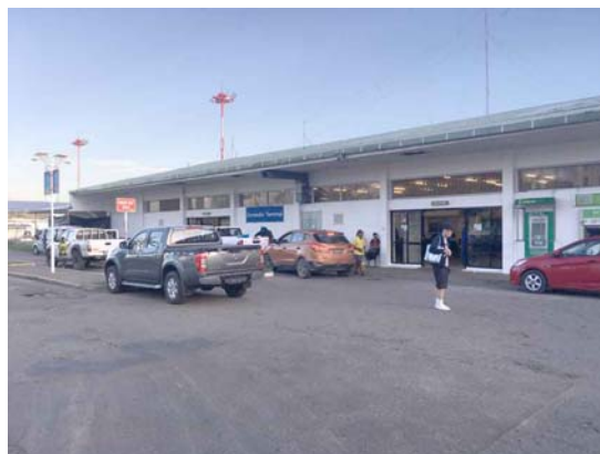
Photo 3.8 Domestic Terminal Building Exterior
