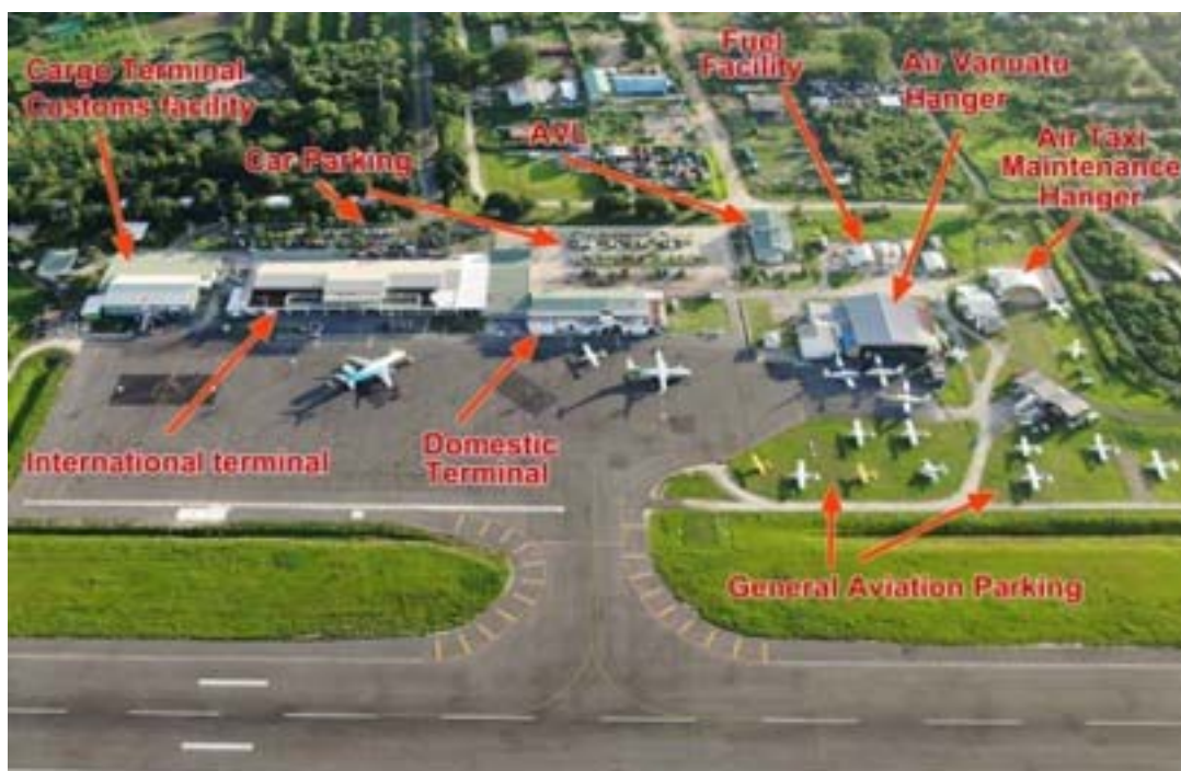
Photo 3.4 Aerial Image of the Existing Terminal Area
