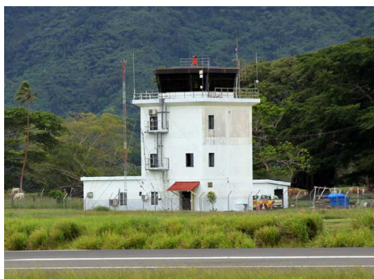
Photo 3.10 Air Traffic Control Tower
