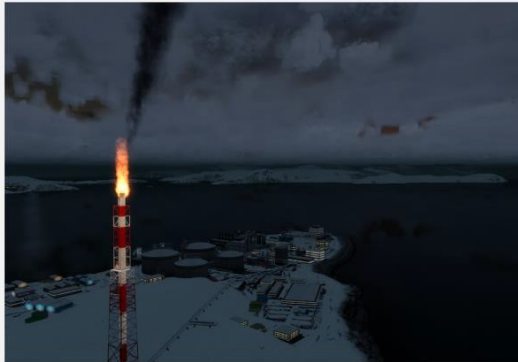
Fire and Smoke
