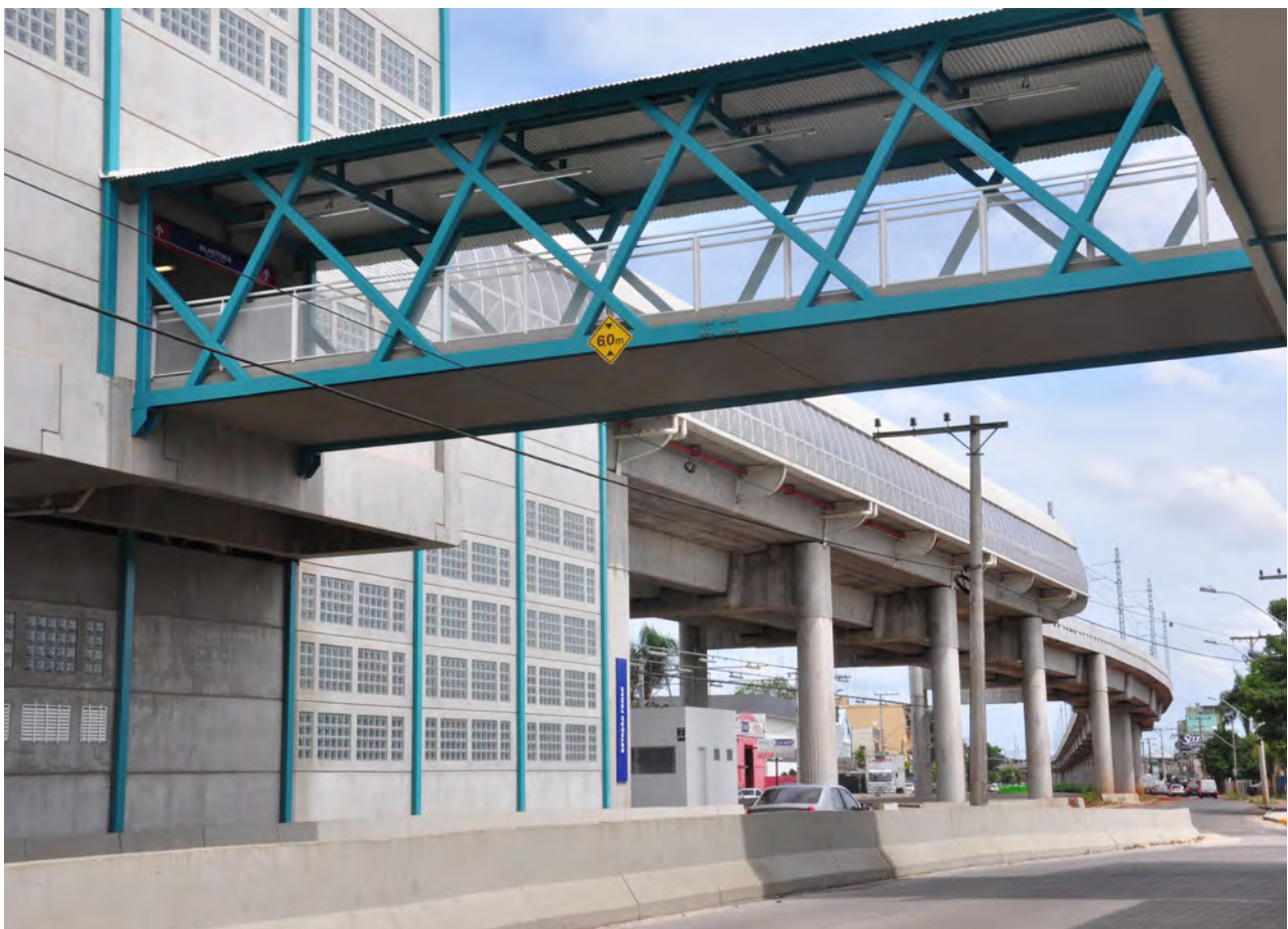
↓ FIGURE - FENAC STATION (TREN SURB), NOVO HAMBURGO.
