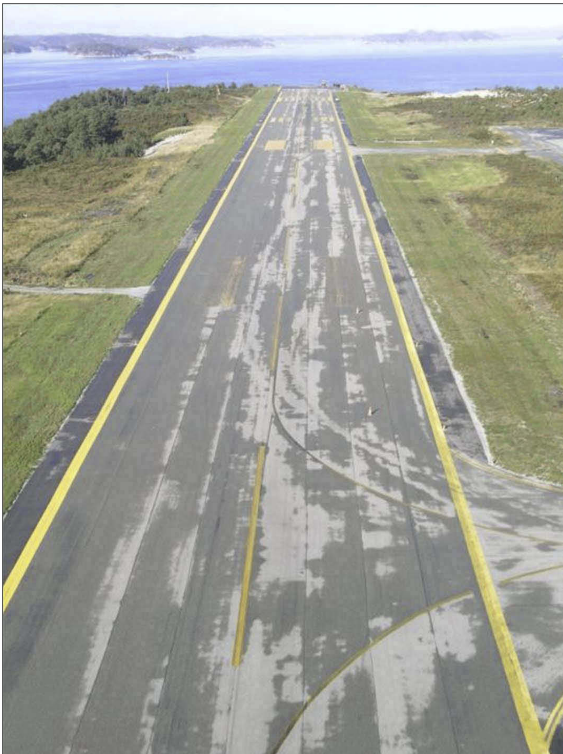
Figure 19: The runway photographed from the helicopter at 1308 hours.
