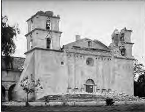
The Santa Barbara Mission was damaged by the 1812 earthquake and rebuilt by 1820. The 1925 earthquake caused the extensive damage shown in this photograph.
