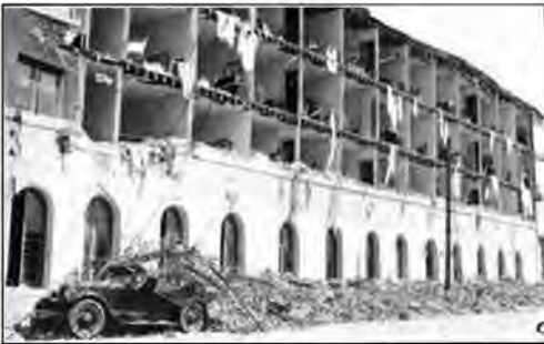
The California Hotel opened four days before the earthquake and experienced heavy damage to brick walls that were not securely tied to the building. Some occupants left the building by lowering themselves to the street using bed sheets.
