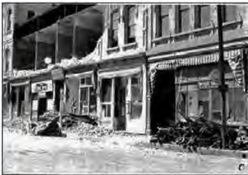
Many of the unreinforced masonry buildings along State Street were damaged or destroyed.
