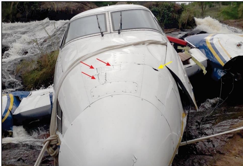
Figure 40 - Contact marks of the cable against the nose of the aircraft. The red arrows point to friction marks, and the yellow arrow shows one of the perforation points in the coating.
