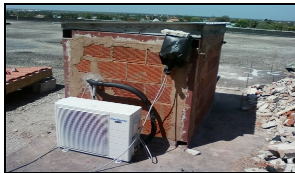
Figure 4. Model 1 - 100mm Clay block walls and corrugated galvanised iron sheeting roof
