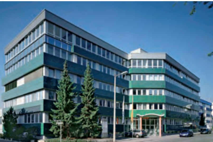
Lapp-Center in Stuttgart
