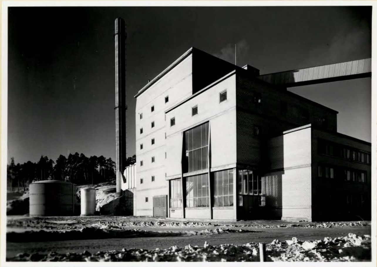
Photograph 1. Exterior of the power-station.
