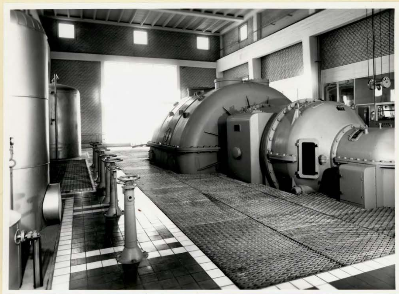
Photograph 2. Interior of the turbine room.
