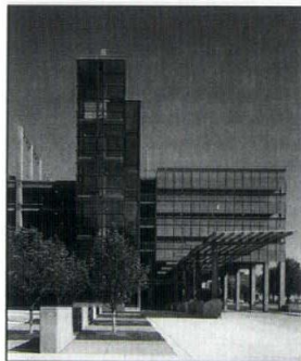
Center Street Park and Ride, Des Moines, Iowa
