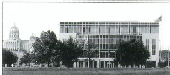
United States Federal Courthouse Annex, Des Moines, Iowa
