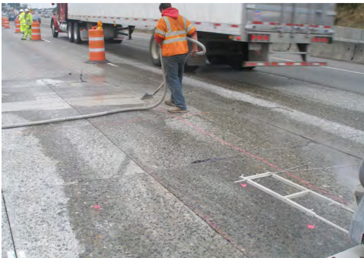
Photo: Pavement repair work Source: Washington State Department of Transportation
