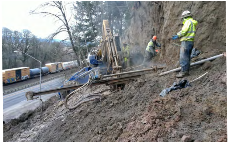
Photo: Landslide repair work Source: Washington State Department of Transportation
