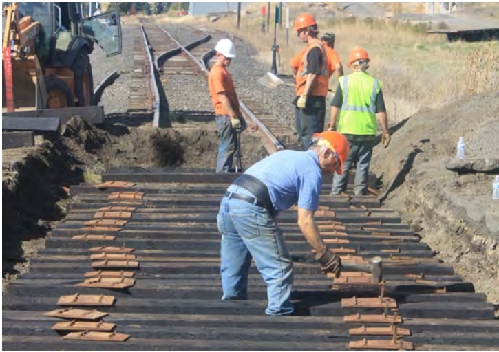
Photo: Railroad maintenance. Department of Transportation
