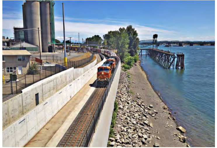
Photo: Rail trench along Columbia River Source: Washington State Department of Transportation
