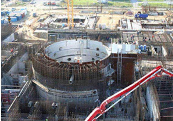
FIG. 37. The sodium cooled fast reactor BN-800 (Russian Federation).
