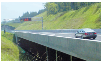
Iron bridge test road simulating highway driving (Toyokoro)
