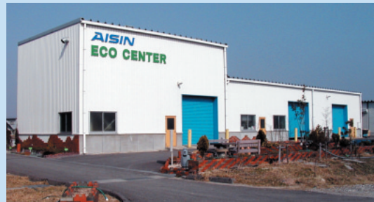
AISIN Eco Center for recycling industrial waste
