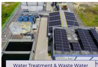
Water Treatment & Waste Water Treatment Plant
