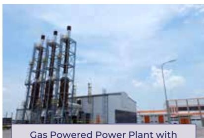
Gas Powered Power Plant with Rooftop Solar Panel
