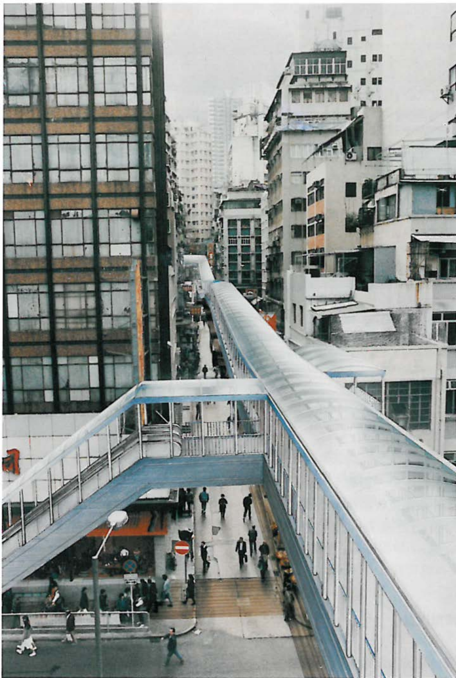
A unique new feature of the 1992 capital works programme is the 800 metre Hillside Escalator Link now nearing completion. The Link rises 135m between Central and the Mid-Levels and is designed to reduce traffic congestion by turning Mid-Level business commuters from motorists to pedestrians. Courtesy the Highways Department.
